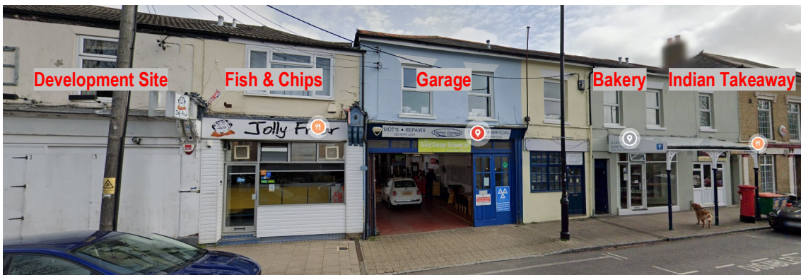
Figure 5.2: The Site and Surrounding Land Uses – View 2
