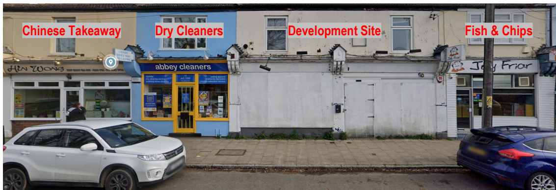
Figure 5.1: The Site and Surrounding Land Uses – View 1
