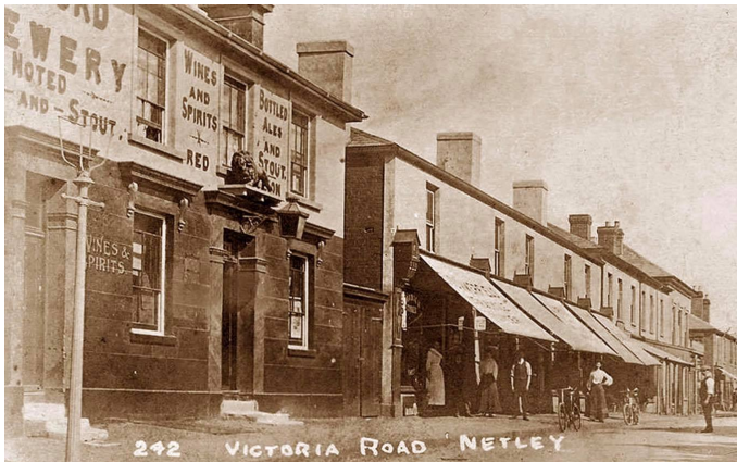
Figure 13: Application Site displaying canopy to frontage
