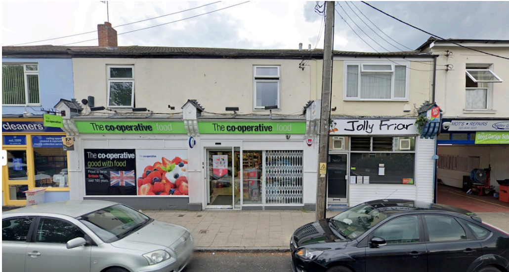
Figure 12: 33, 34, 35 Victoria Road showing removal of historic entrances
