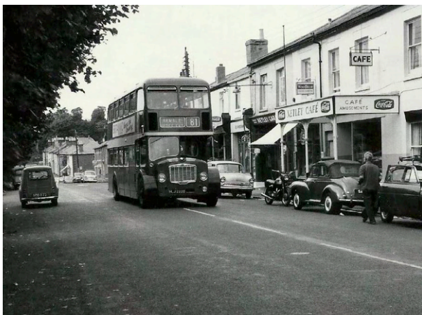
Figure 15: Application Site looking eastwards
