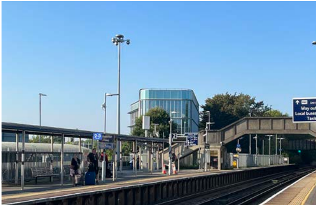
External view from Southampton Parkway railway station
