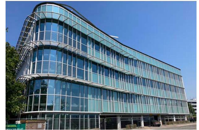
External view of main elevation to Mitchell Way
