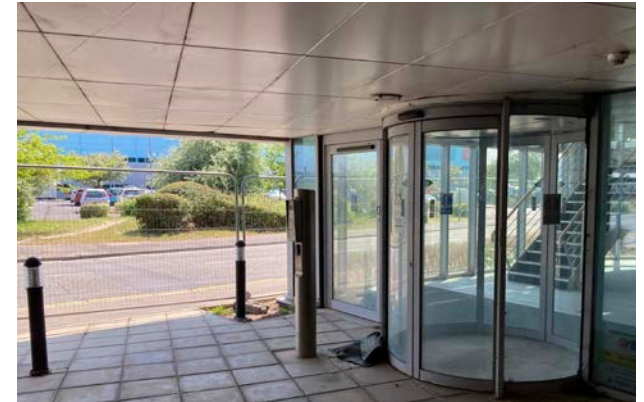
Exterior view of main entrance off undercroft parking
