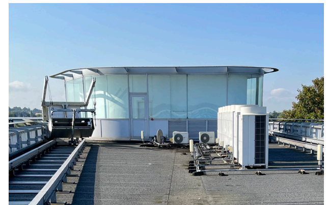
External view of flat roof cupola (plant room)
