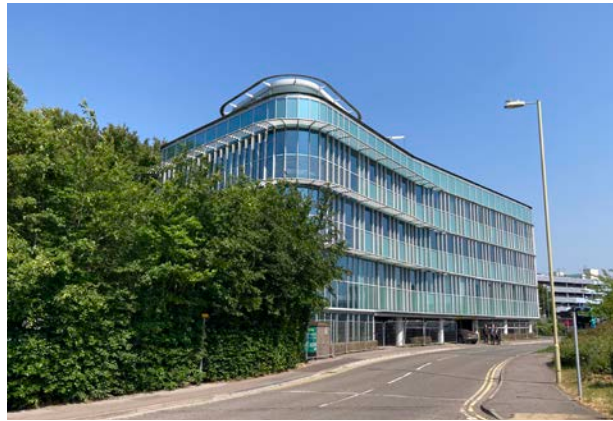
External view north on Mitchell Way
