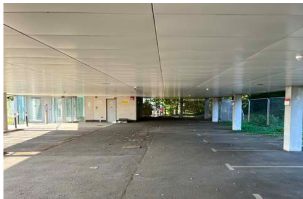
Exterior view of undercroft car park
