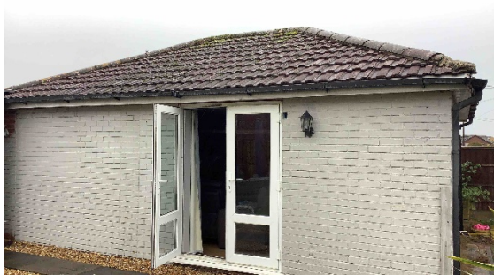
Photograph 1. B1 former garage.
