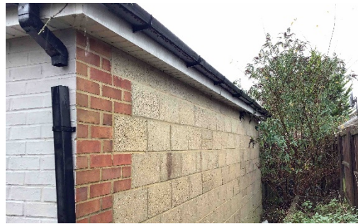
Photograph 2. B1 former garage.
