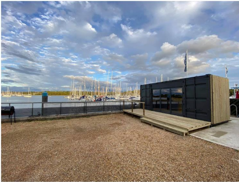
Figure 1: Former WeSUP Site
