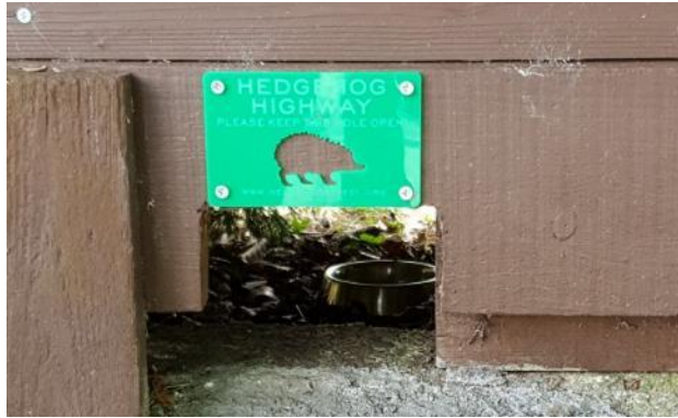
Figure 27. Example of permeable garden fencing (Source: Hedgehog Street Website)
