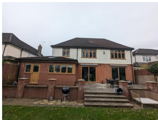
Figure 4. Eastern elevation of the property (rear)
