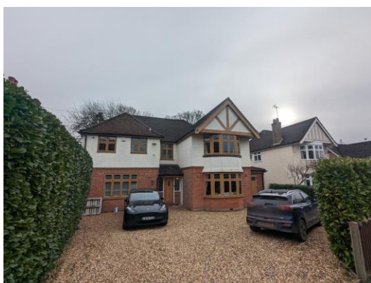
Figure 2. Western elevation of the property (front)
