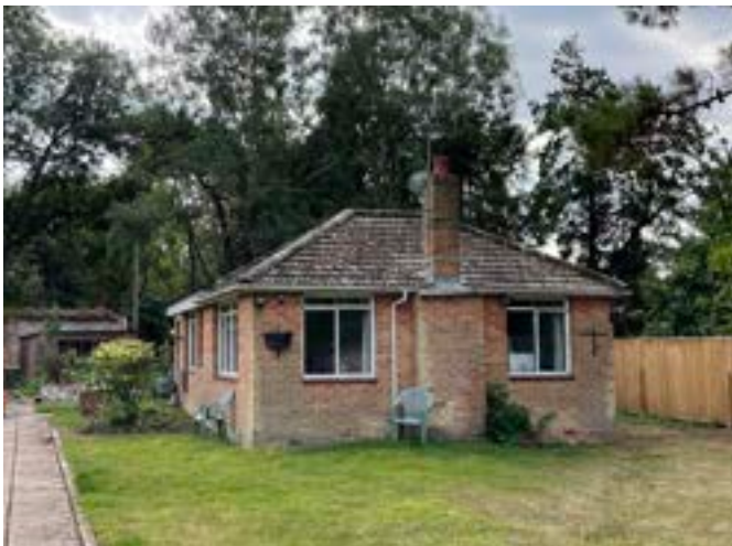
Existing bungalow in disrepair
