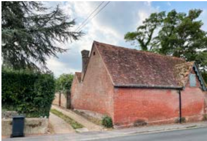
The existing site access that will serve Plot 1.
