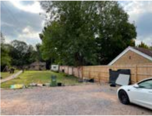
5 - The western half of the southern boundary wall collapsed and has been replaced with fencing, maintaining the boundary between the two properties.
