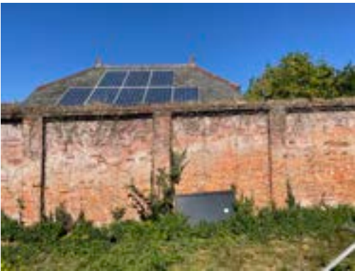
1 - The segment of wall to the north-west of the site appears in reasonable condition, forming a barrier between the site and the properties to the north. This wall lies outside of the site boundary.
