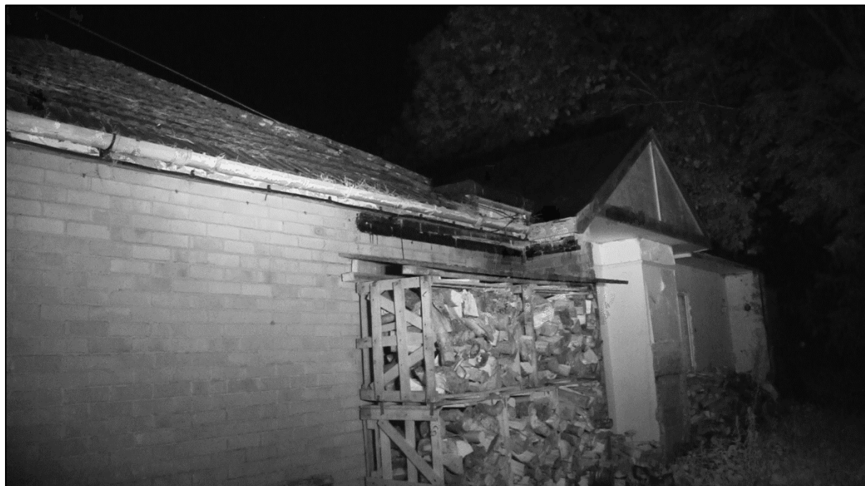
Figure 2 – Infra red at end of survey – South, West and North Elevations
