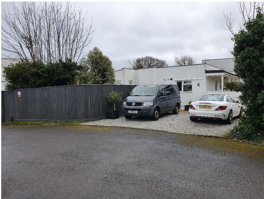
Fence and pedestrian gate section (6.75m) adjacent to off road parking at the side of 4 Crowsport, reinstating security and privacy for rear garden.
