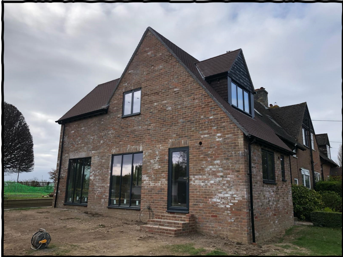
Similar Approved and BUILT Extension at 7 Knowle Lane
