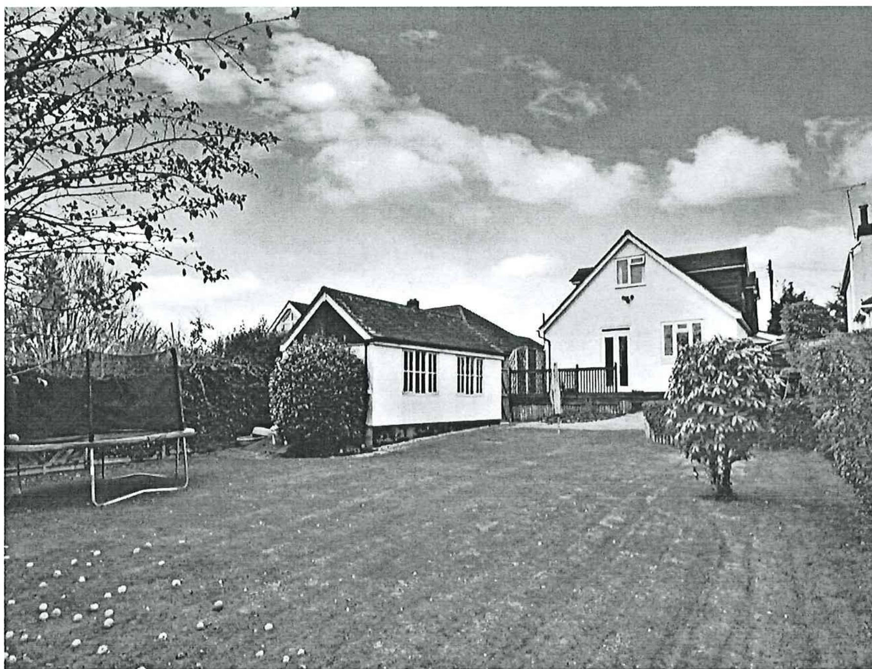
NORTH FACING DORMERS (R) FACING 40 YARDLEY ROAD THE FURTHEREST TWO ARE CLEAR GLAZED , THE NEAREST ONE IS BELIEVED TO CURRENTLY BE OPAQUE AS IT IS A BATHROOM
