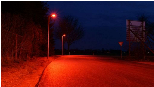
Figure 8: Bat friendly red street lighting.
