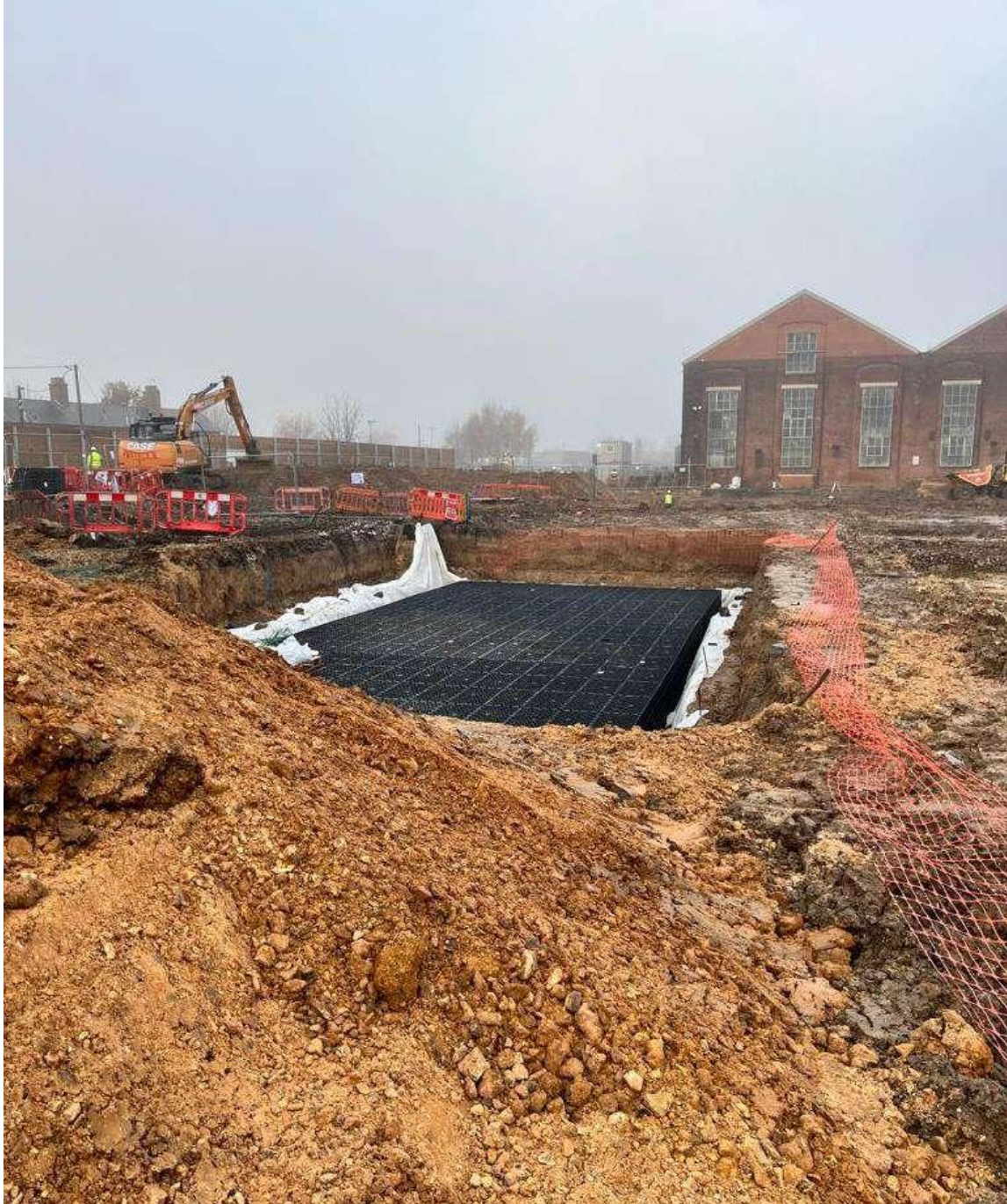
Figure 10 – Watching brief during drainage & service ducts.
