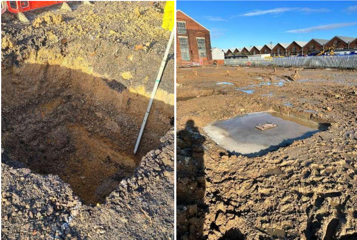
Figure 8 – Watching brief during groundworks.
