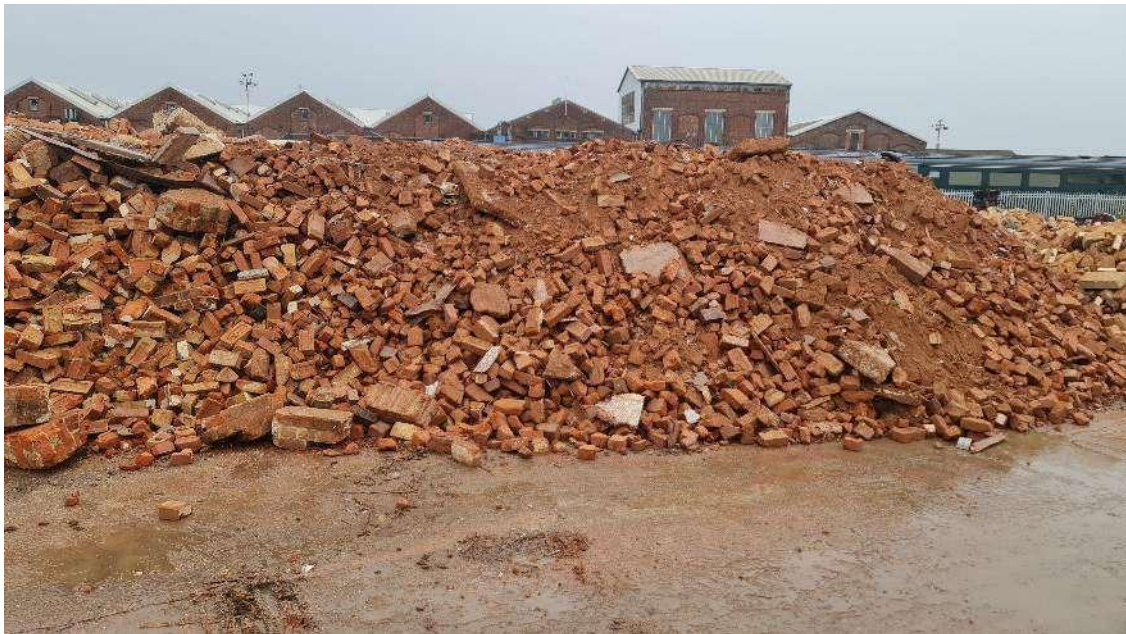
Figure 5 – Demolition Stockpile (prior to crushing).
