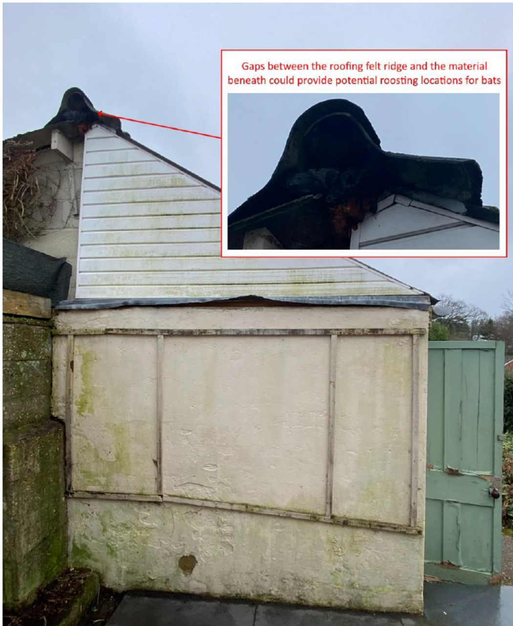
Image 4.3.2.1. Location of potential bat access points on the west elevation of the shed.
