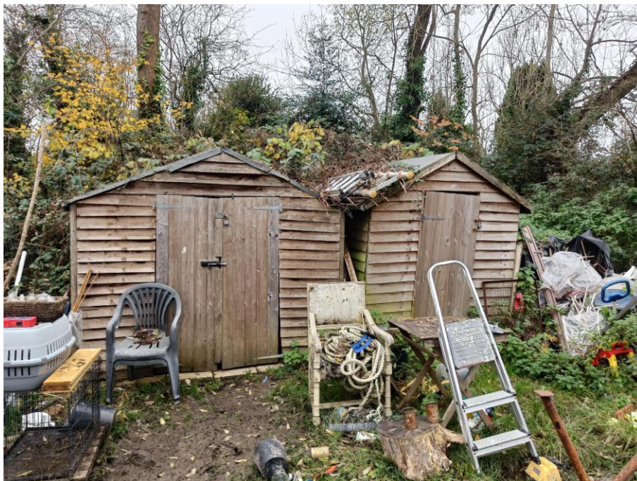
Figure 8. View of the sheds present on site (taken November 2023).
