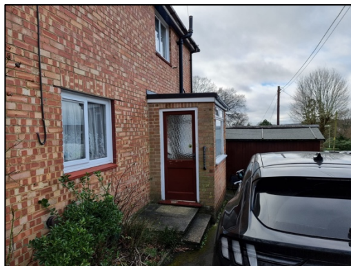
Figure 3 – western elevation with single extension
