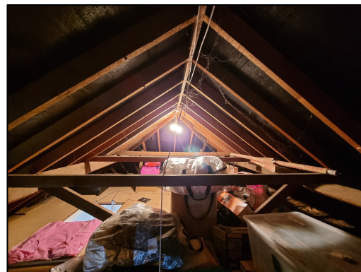
Figure 4 – interior roof void of the house
