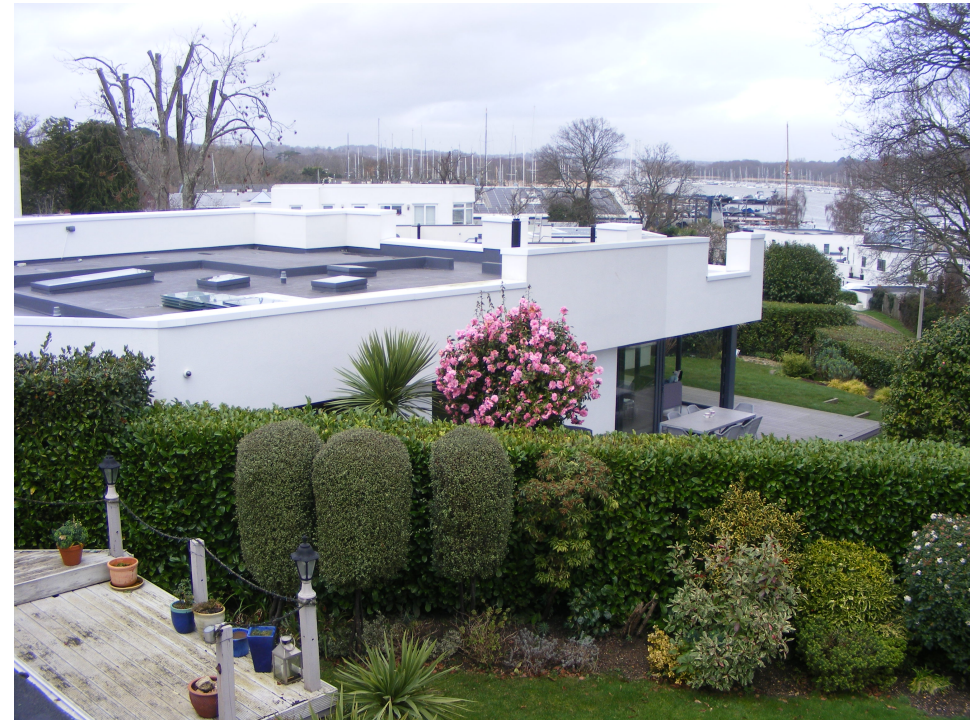
(02) Photo looking North towards No.16, highlighting the extent of viewing that could be achieved from the unscreened end of the new proposed new Roof Terrace, located outside to the new Master Bedroom.
