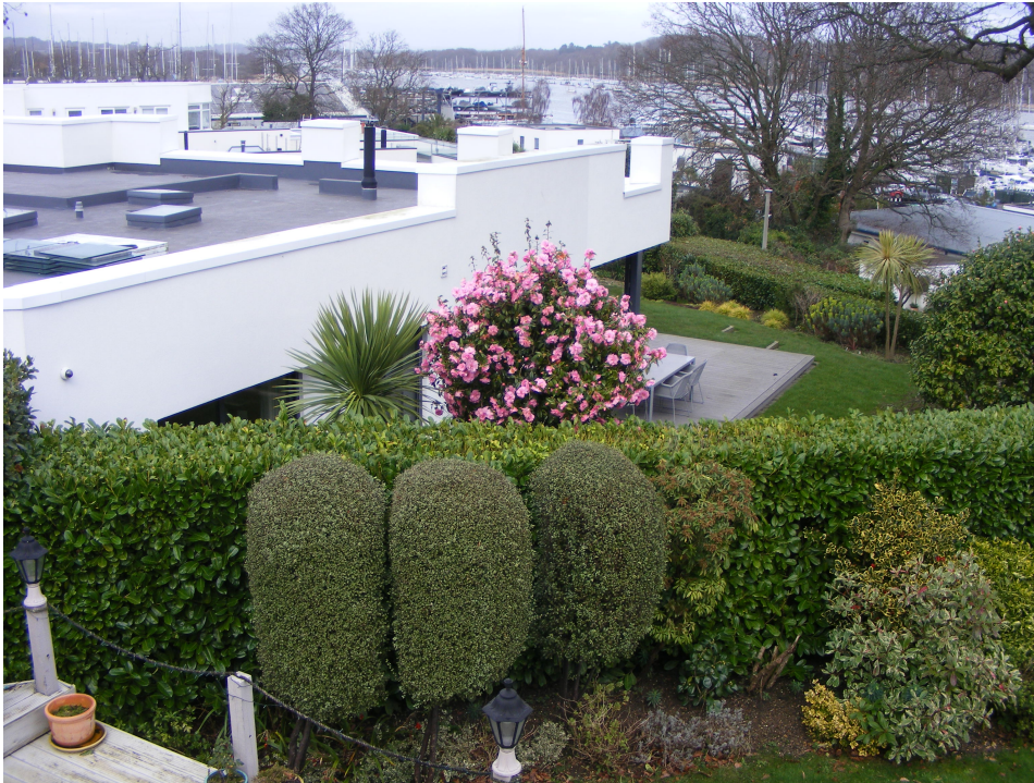
(01) Photo looking North from the roof of No.15 Crowsport, highlighting the nature of the existing Boundary between No.15 and M.16 Crowsport Estate, taken from the location due to be protected with Visibility Screening on top of a 1.1m high parapet Roof Terrace wall.
