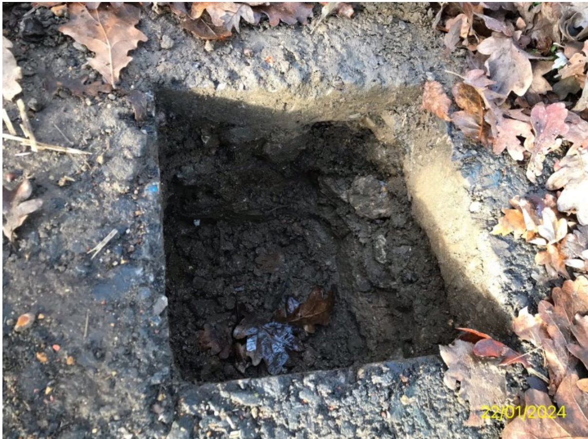
Image 5: Trial Hole 4 tarmac layer and below this was a single layer of stone hardcore, the geotextile membrane is not visible in this photo because of soil that has buried it over time. Trial hole 4 is visually similar to trial hole 1.
