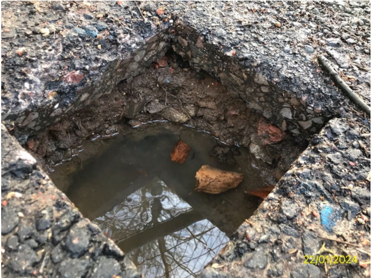
Image 3: Trial Hole 2 tarmac layer and below this was a single layer of stone hardcore, the geotextile membrane is not visible in this photo because of the water.
