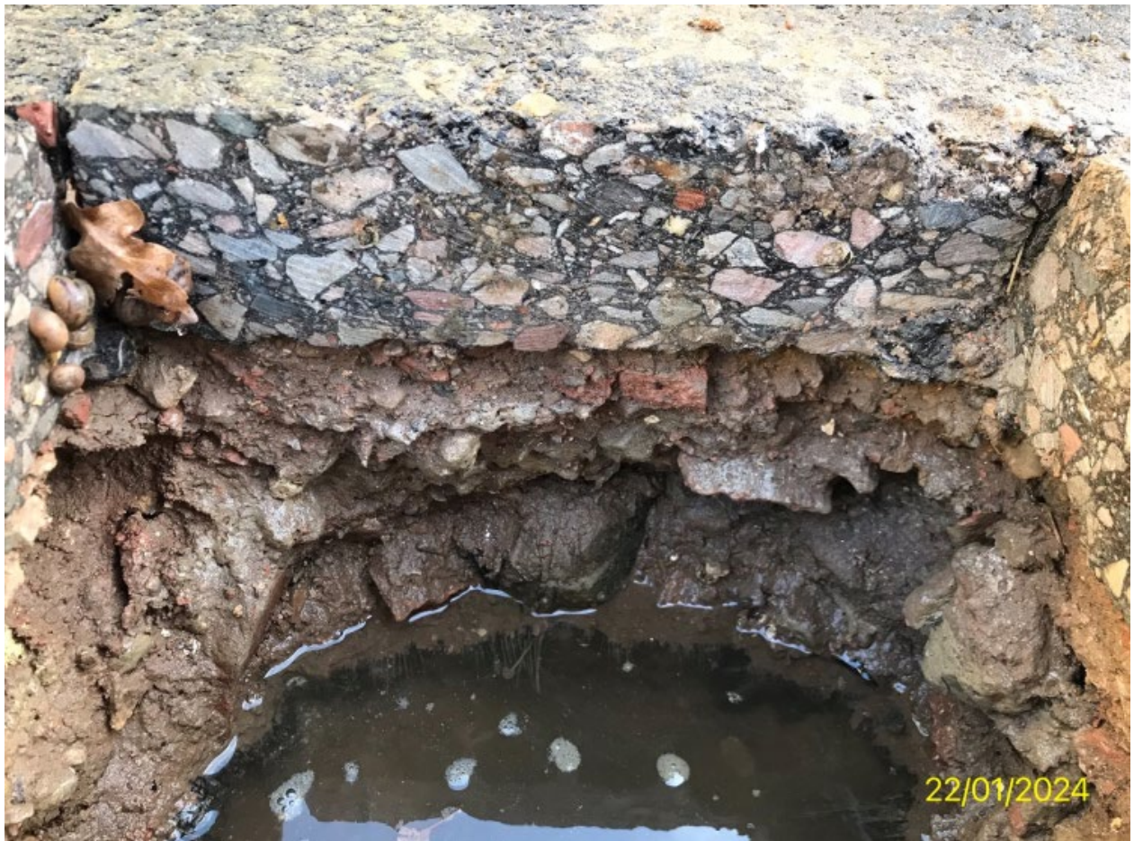
Image 2: Trial Hole 1 – tarmac layer and below this was a single layer of stone hardcore, the geotextile membrane is visible in this photo just below the waterline.
