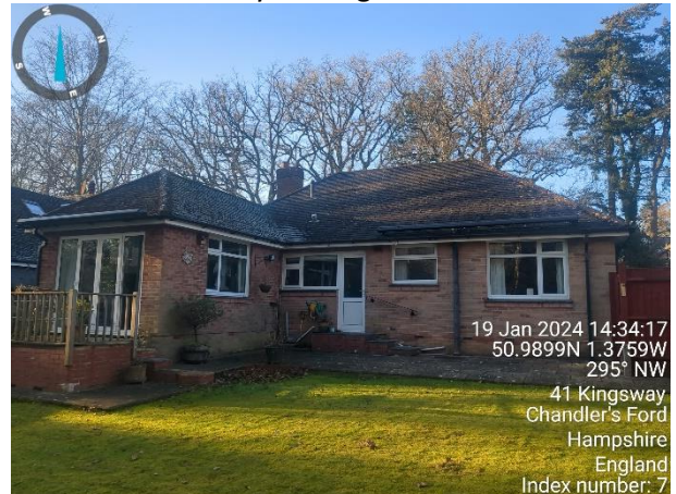
Photograph 12: View of the bungalow from the rear.
