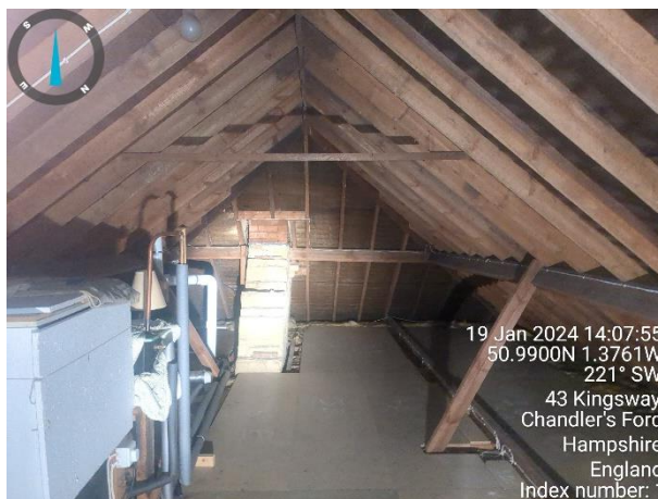
Photograph 23: View within the bungalows loft looking south.
