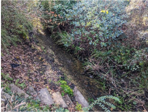
Photograph 7: View of the wet ditch and the steep embankments.
