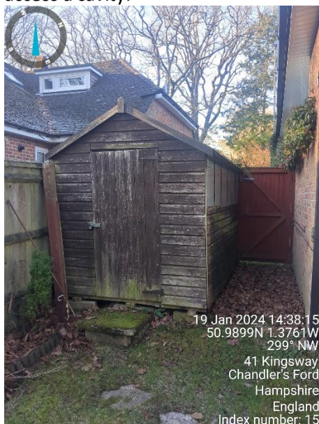
Photograph 17: View of the shiplap shed on the southern boundary.
