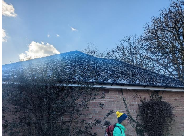
Photograph 2: View of the north-west elevation roof.
