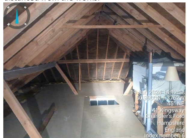
Photograph 24: View within bungalows loft looking north.
