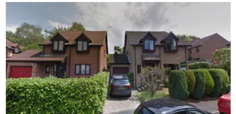
54 Eden Road - 2 Storey 80s Link Detached Houses
