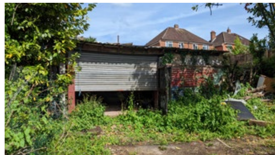
VIEW 3 - Existing garage entrance
