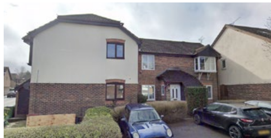
18 Hayle Road - 2 Storey 80s Terraced Houses
