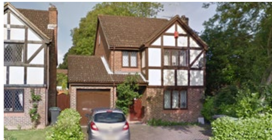
39 Eden Road - 2 Storey 80s Detached Houses
