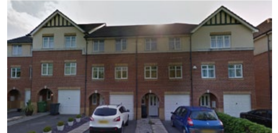
88 - 94 Eden Road - 3 Storey 00's Town Houses
