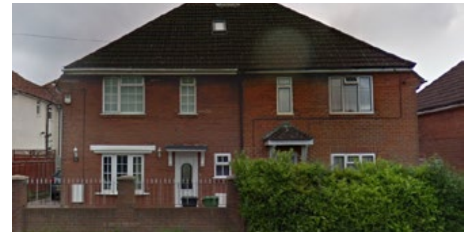
65-67 Swaythling Road - 2.5 Storey 70s Semi-detached Houses
