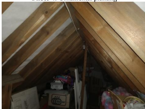
Photo 6: Roof void, main house
