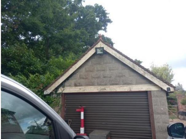
Photo 7: Northern elevation of garage
