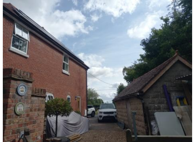
Photo 8: Southern elevation main house, and northern and western elevations of garage
