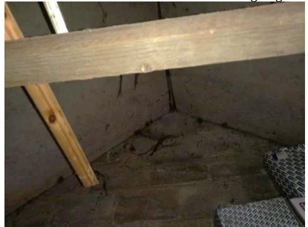
Photo 10: Roof void within garage
