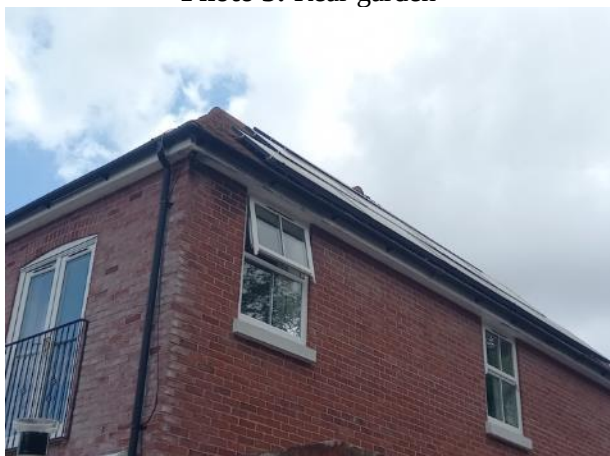
Photo 5: Roof detail, eastern elevation, main house
