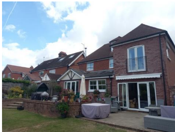
Photo 2: Rear (western) elevation of main house
