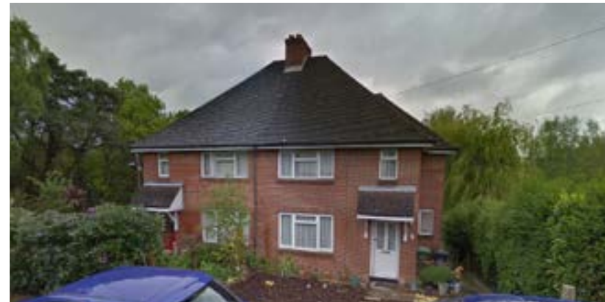
17-18 PEEWIT HILL – 2 STOREY 80s SEMI-DETACHED HOUSES
