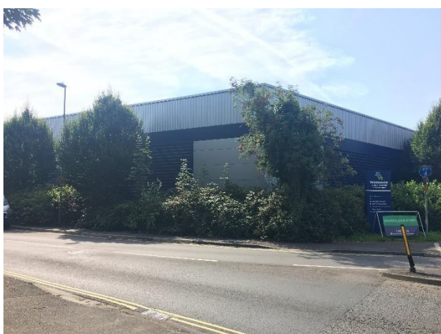
Figure 6: Existing North elevation of the unit
