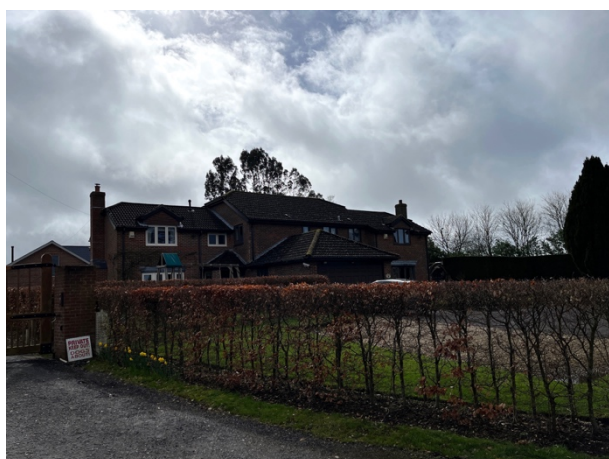
The barn-hipped roof of 'Corringham House'.
