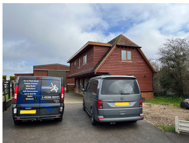
The subject building, viewed from the southwest.
