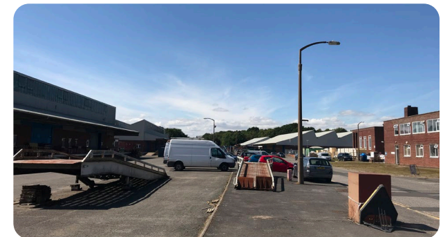
The central estate road access to Chalcroft Business Park
