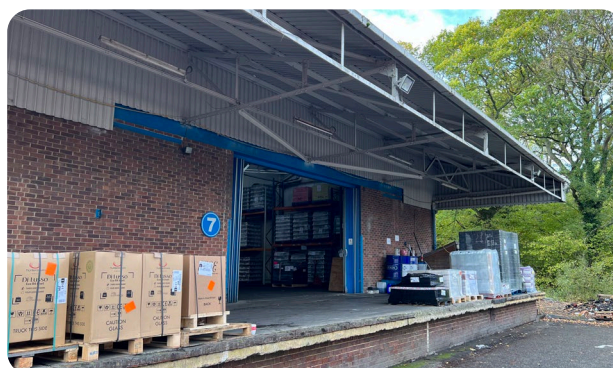
Unit 7 - brickwork and steel structure frame
