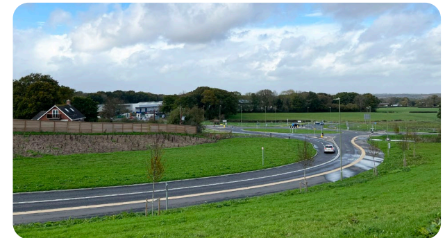
The new link road - Chalcroft Way
