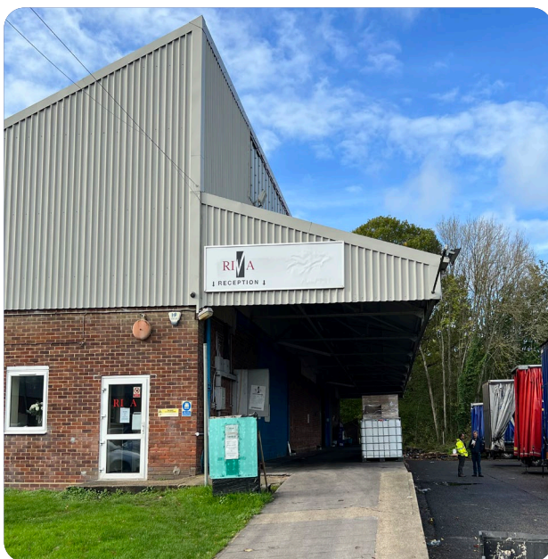
Loading area to existing commercial unit
