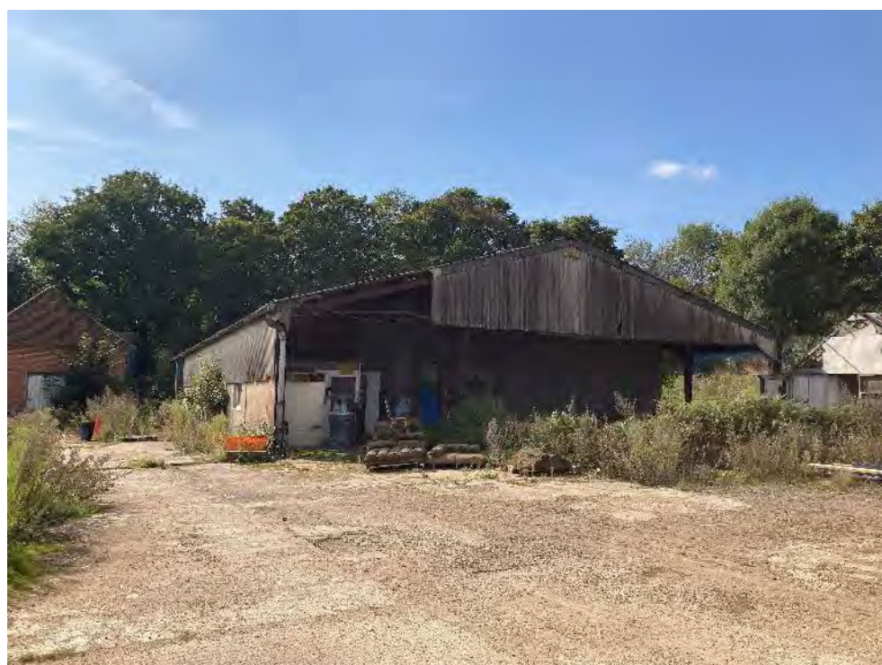
Photograph 6: View of the former farm buildings and hardstanding in the north-western part of the site, looking north-west.
