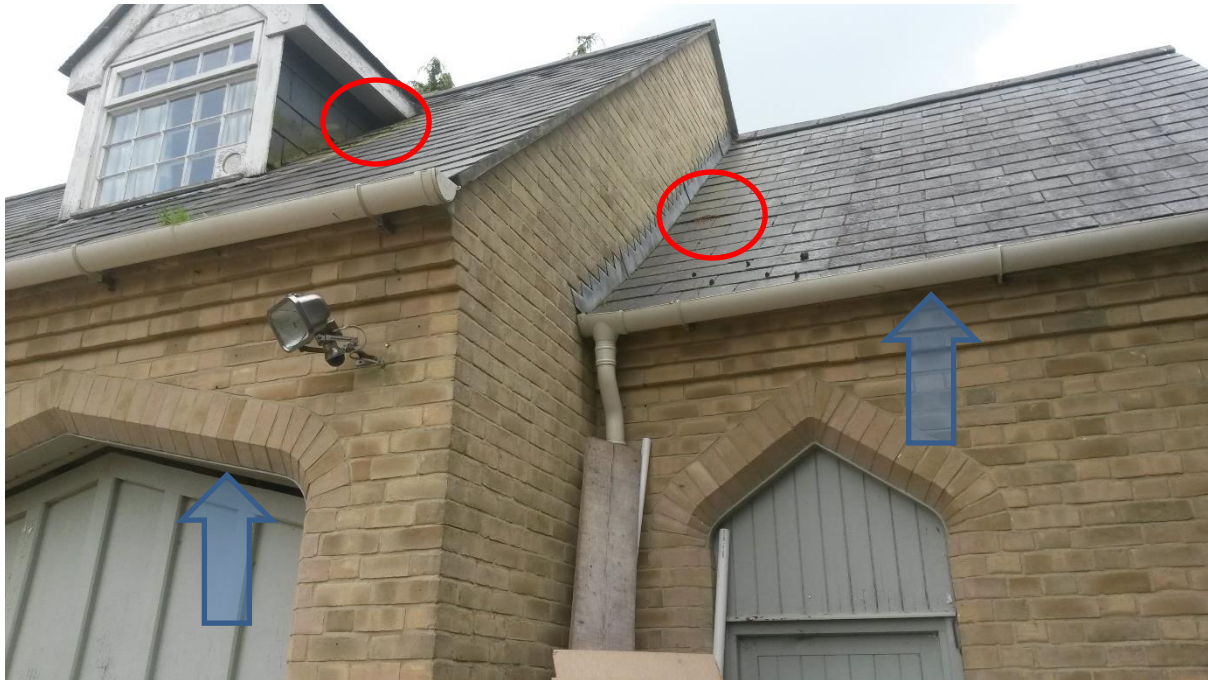
Photo 3: Close up view of section being demolished and potential access under slate and at dormer window. Potential access points are also present under the guttering leading into the attic area. The gap above the attic door is also visible in the photo.
