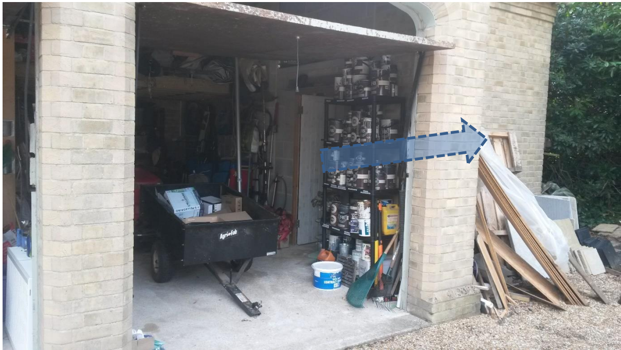
Photo 7: Bat access through door into store area and then outside via garage door (either open or closed)
