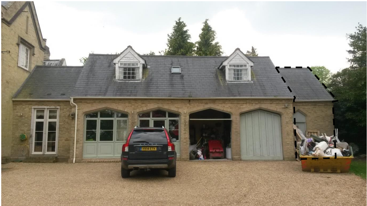
Photo 2: The garage section, the room being demolished is on the right hand side of the photo
