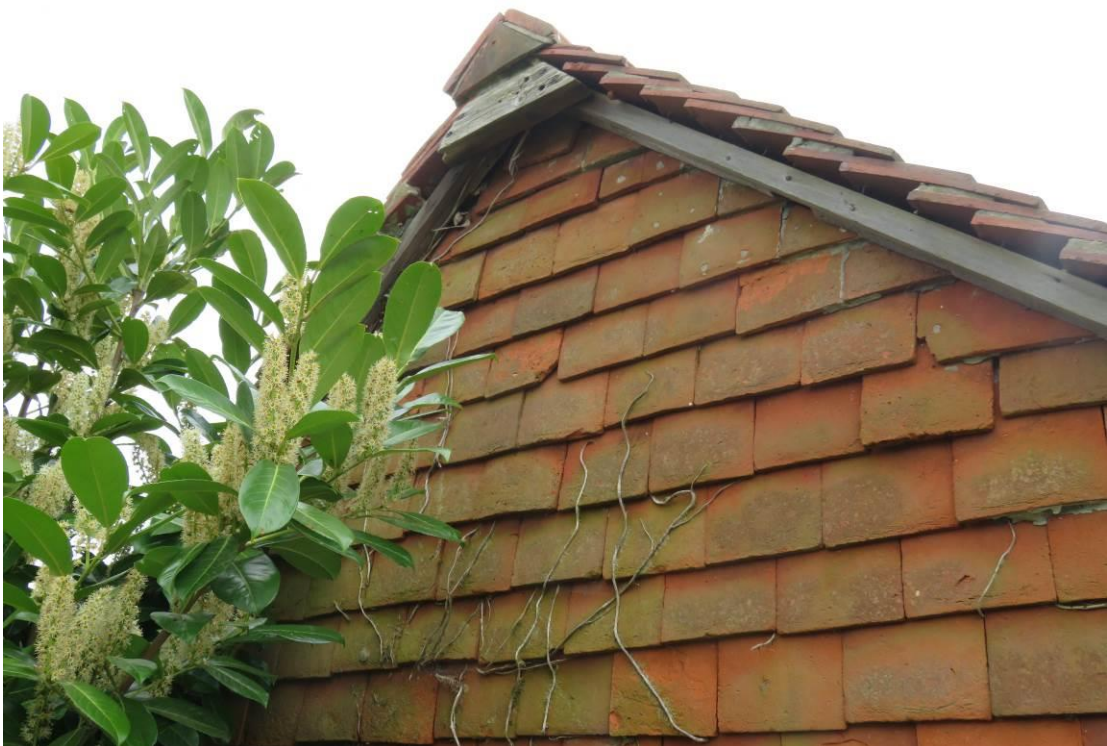
Photo 11/12 Ancillary – moderate potential , no recorded use to date, building retained.
