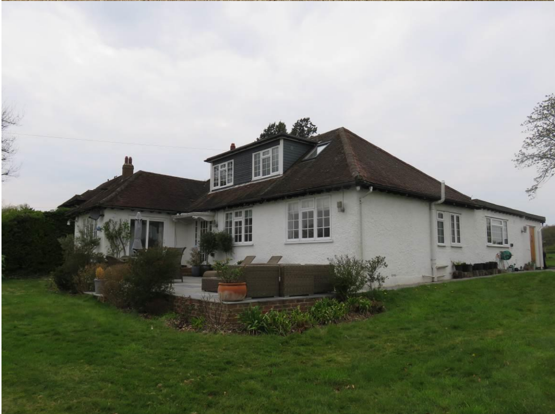
Photo 1/2 Badnum Cottage (North and south aspect), Current bat roost locations.
