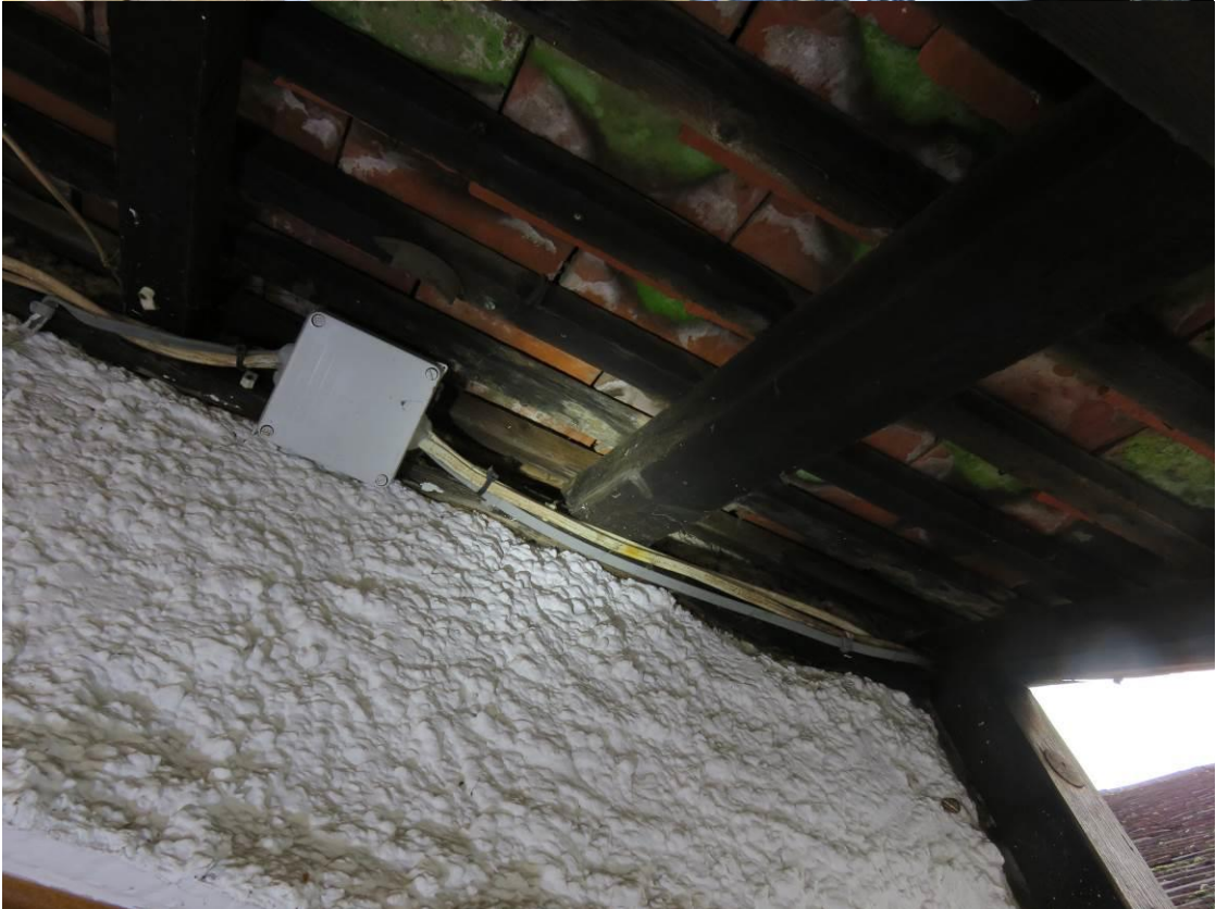
Photo 9/10 Roof void areas . No. Dropping evidence recorded.
