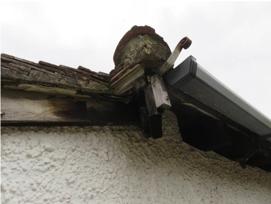
Photo 5/6 Badnum Cottage roof details
