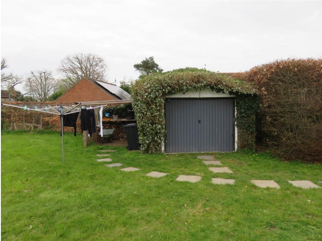
Photo 15 Modern Garage , no recorded use to date, building retained.
