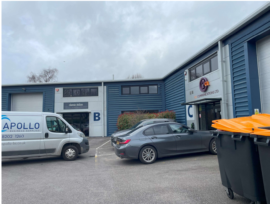
Unit C, Woodside Trade Centre – site photographs 13/03/2024 App ref. F/24/96975
