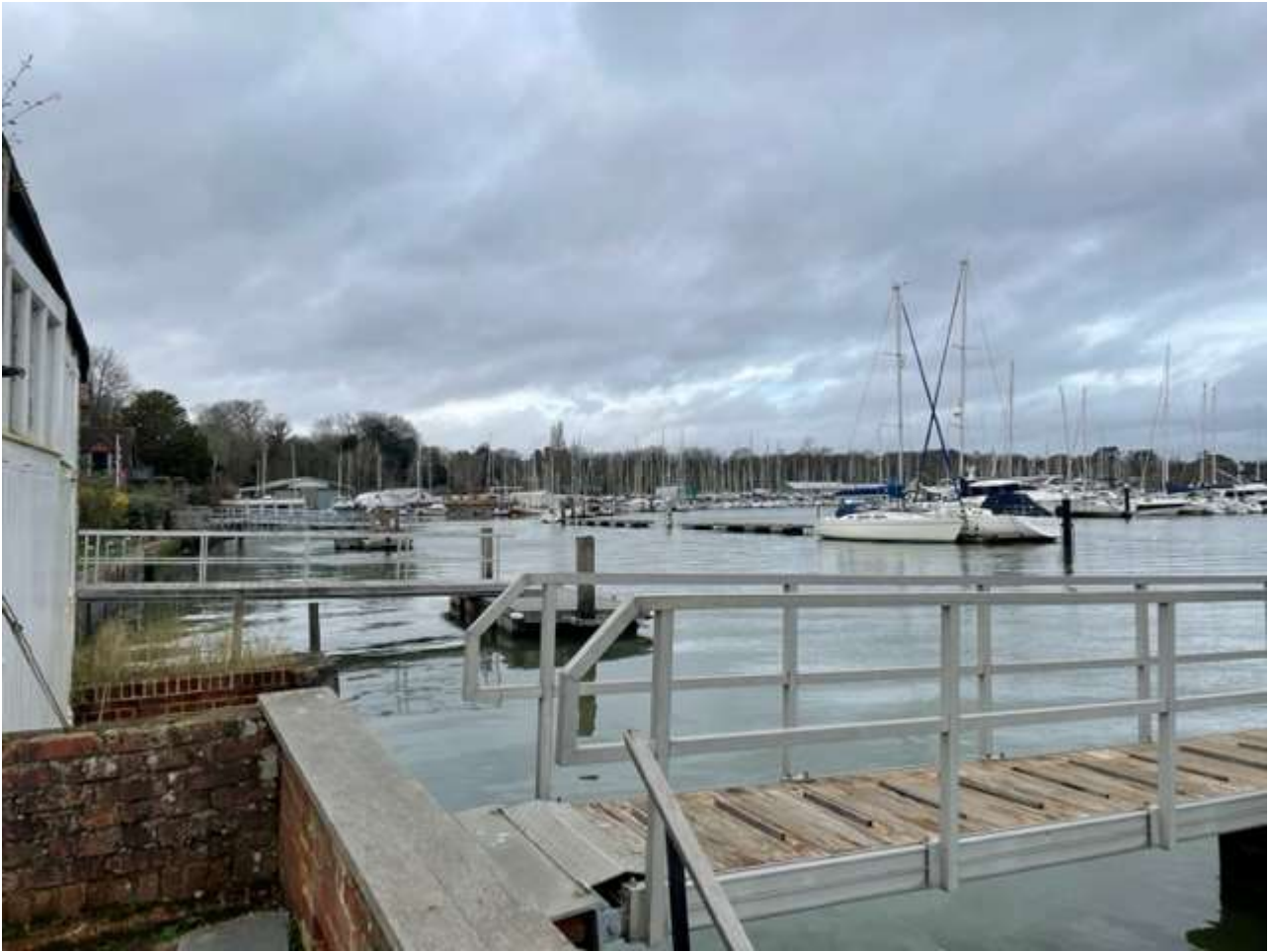
View north west from Lands End House showing existing pontoons.
