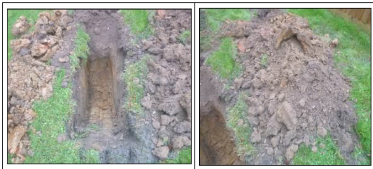
Photograph 8 Trial pit and removed soil material - Location TP.08
