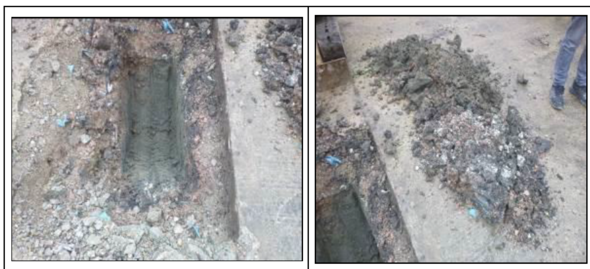
Photograph 7 Trial pit and removed soil material - Location TP.07
