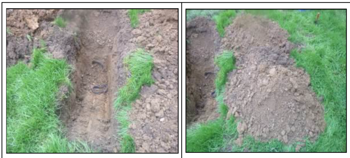
Photograph 10 Trial pit and removed soil material - Location TP.10
