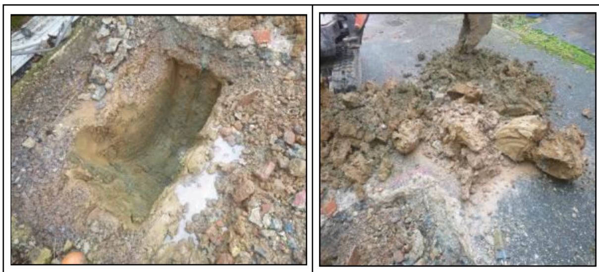
Photograph 5 Trial pit and removed soil material - Location TP.05
