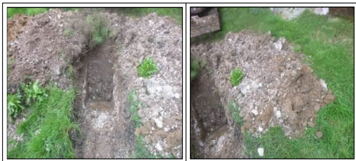
Photograph 11 Trial pit and removed soil material - Location TP.11
