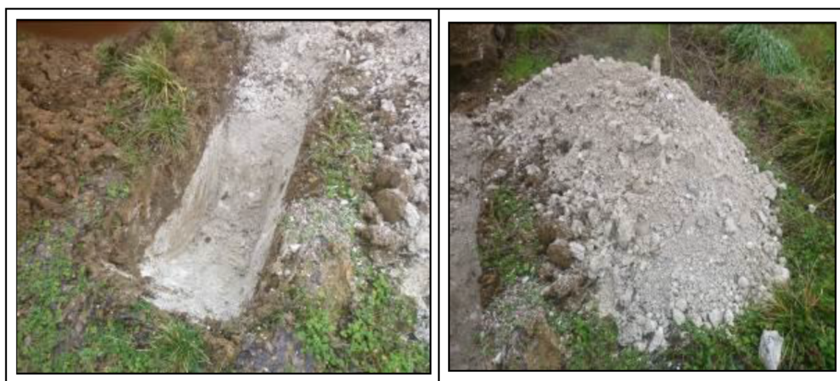
Photograph 12 Trial pit and removed soil material - Location TP.12
