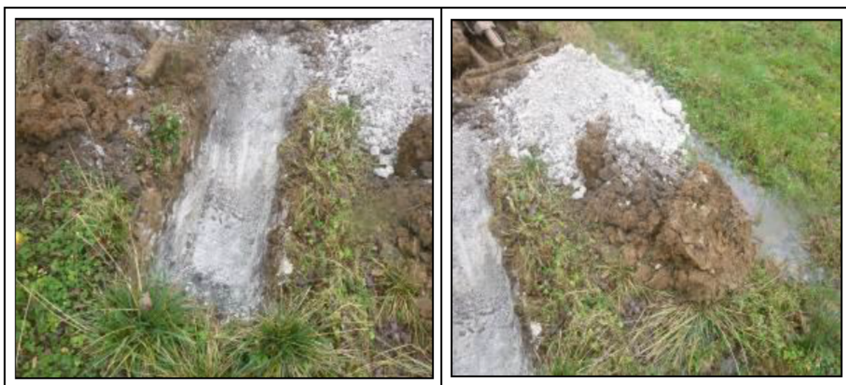
Photograph 13 Trial pit and removed soil material - Location TP.13
