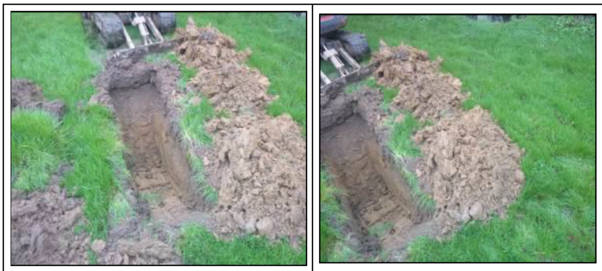
Photograph 9 Trial pit and removed soil material - Location TP.09
