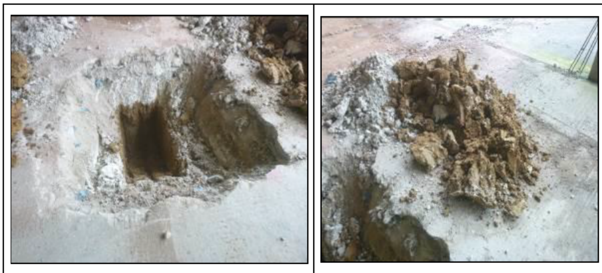
Photograph 4 Trial pit and removed soil material - Location TP.04
