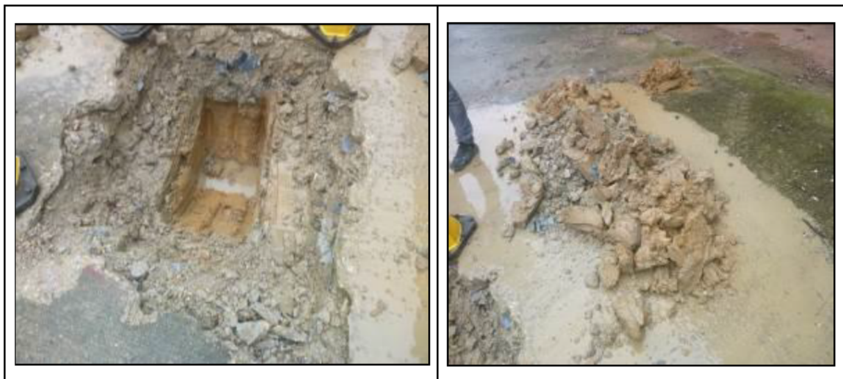
Photograph 3 Trial pit and removed soil material - Location TP.03
