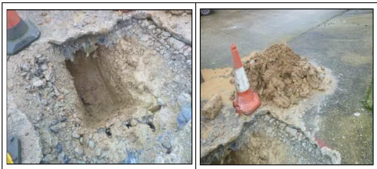
Photograph 2 Trial pit and removed soil material - Location TP.02
