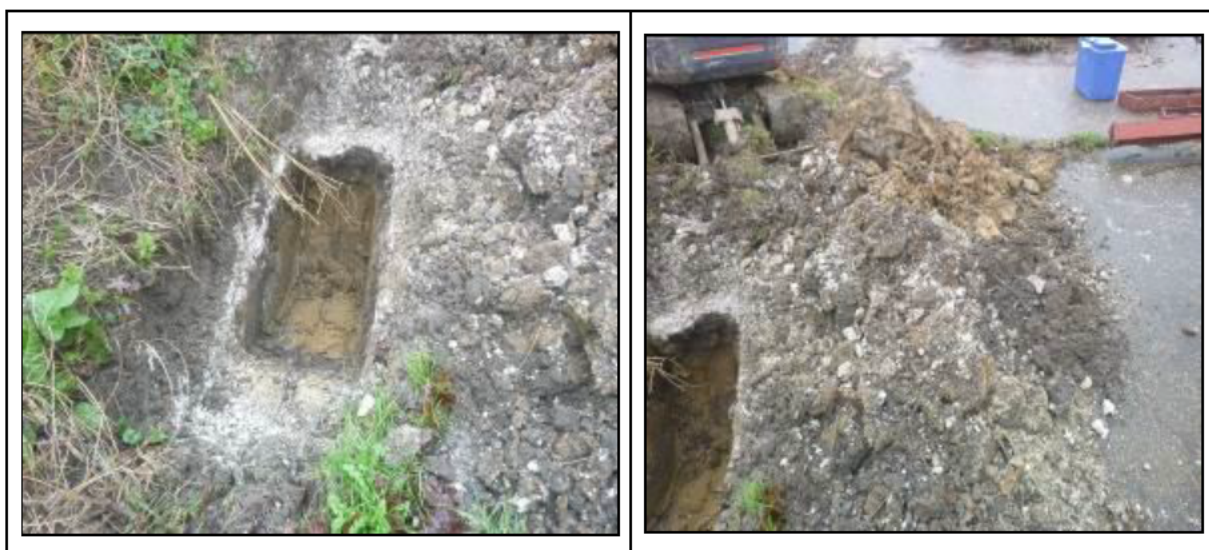
Photograph 14 Trial pit and removed soil material - Location TP.14
