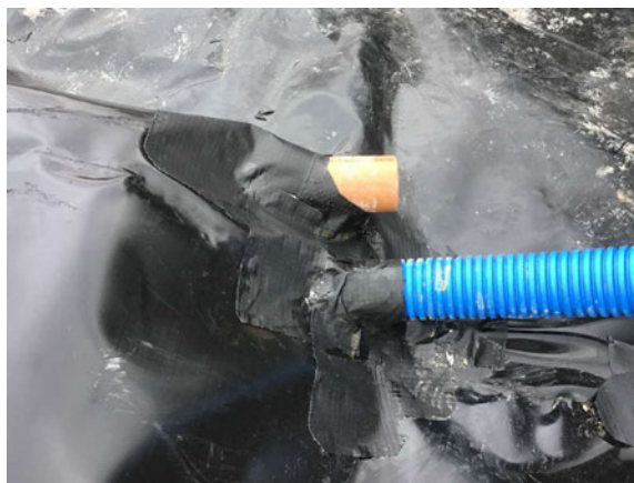
Typical double pipe penetration seal using SAGM.
