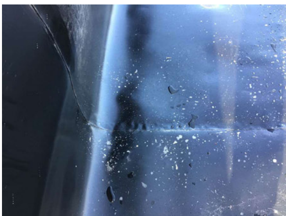
Typical hand welded membrane lap.
