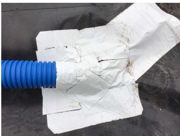
Sealed pipe penetration using SAGM.
