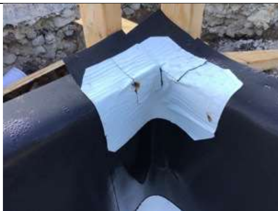
Sealed corner detail using SAGM.
