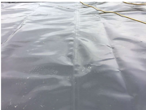
Auto welded membrane lap.
