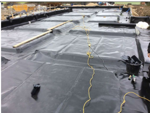
Overview of installed Juta GPH 0.6 gas membrane across the full footprint of unit D.
