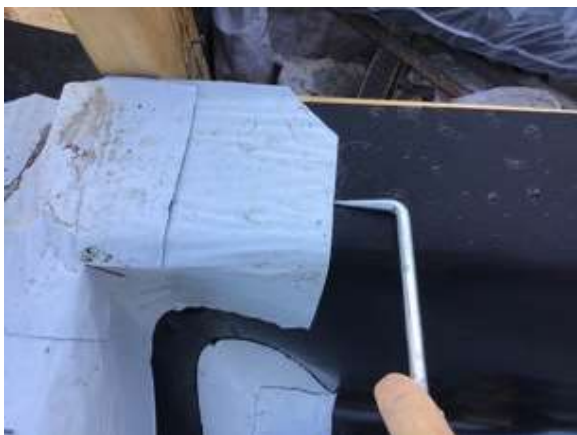
Pick testing all SAGM detailing.
