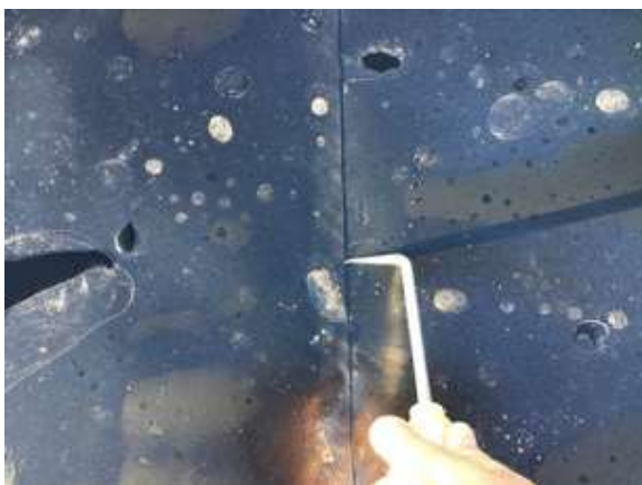
Pick testing all hand welded membrane laps.
