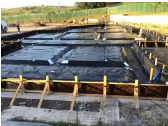
Overview of installed membrane to industrial unit block A.
