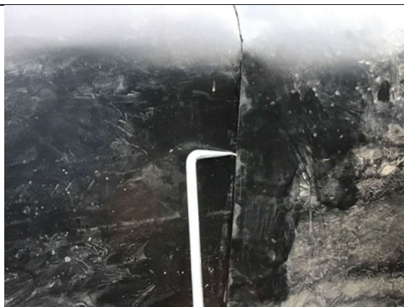
Pick testing all hand welded membrane laps.
