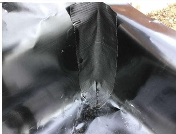
Sealed corner detail using SAGM.
