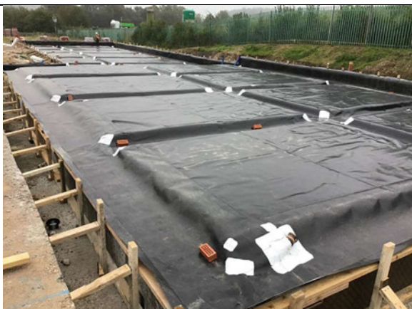
Overview of installed membrane to block E.
