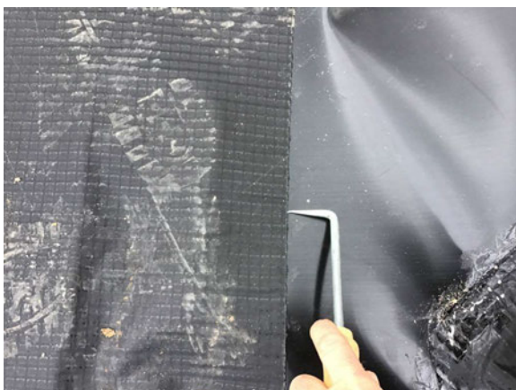
Pick testing all SAGM detailing.
