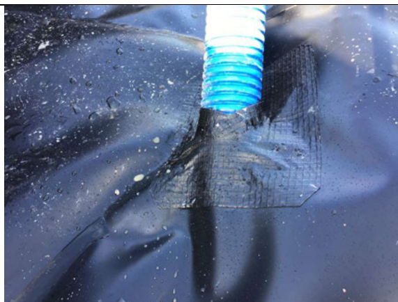
Typical pipe penetration seal using SAGM in block B.
