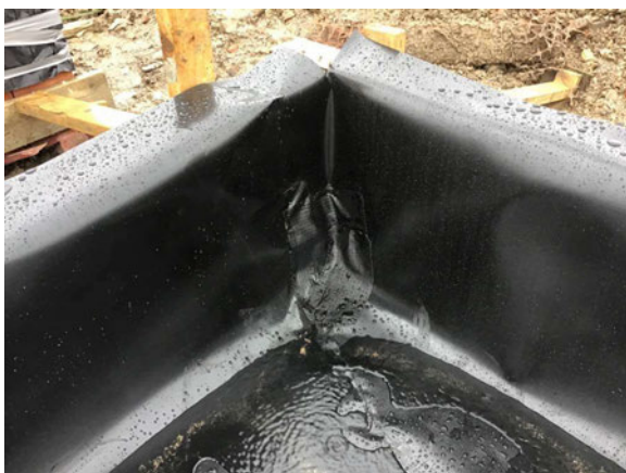
Sealed corner detail using SAGM.
