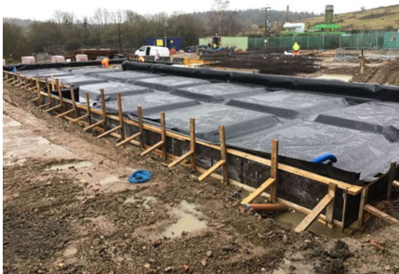
Overview of installed Juta GPH 0.6 gas membrane across the full footprint of unit C.
