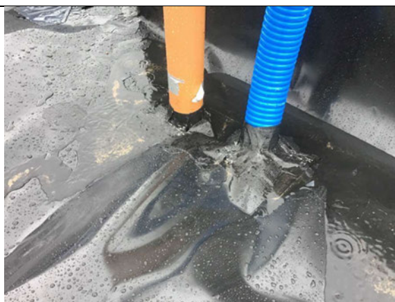
Typical double pipe penetration seal using SAGM.
