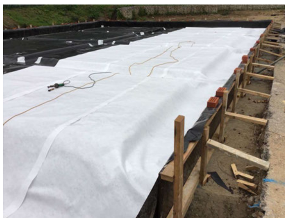
Protection fleece being installed on top of the membrane.
