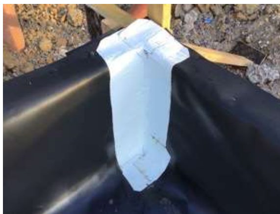
Typical corner seal using SAGM.
