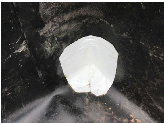
Sealed corner detail using SAGM.
