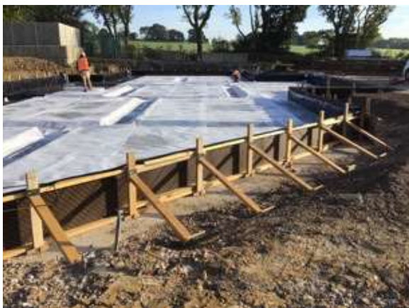
Protection fleece installed on top of the membrane.
