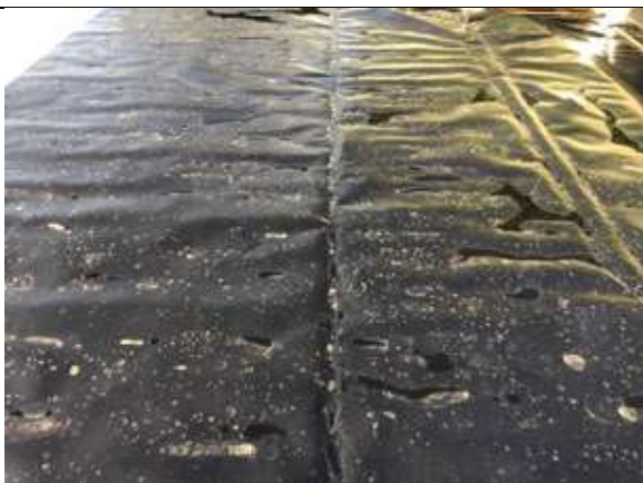
Typical hand welded membrane lap.
