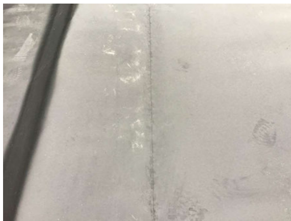
Typical hand welded membrane lap.
