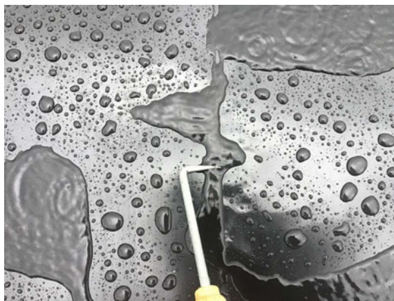
Pick testing all hand welded membrane laps.
