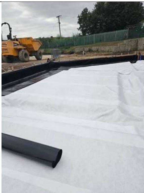
Protection fleece installed under the installed membrane.
