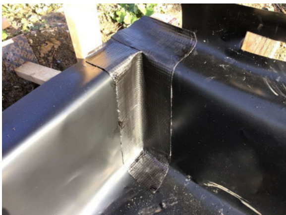
Typical corner seal using SAGM in block B.
