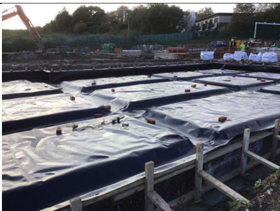
Overview of installed membrane in block B.
