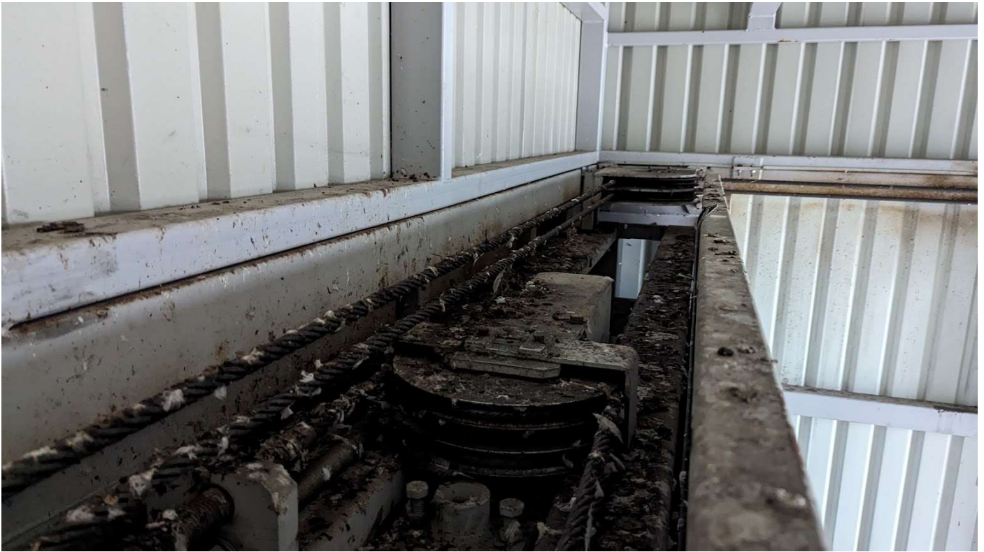
Photo 3 – High level view of the loading bay, showing ledge previously used by birds but with no evidence of nesting.
