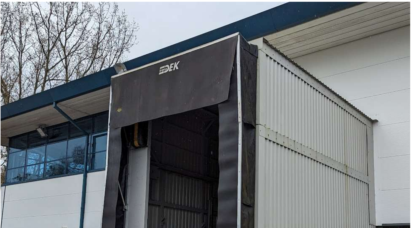
Photo 2 – View of a loading bay.
