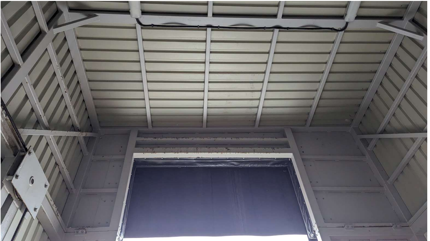
Photo 1 – View inside the loading bays from ground level.
