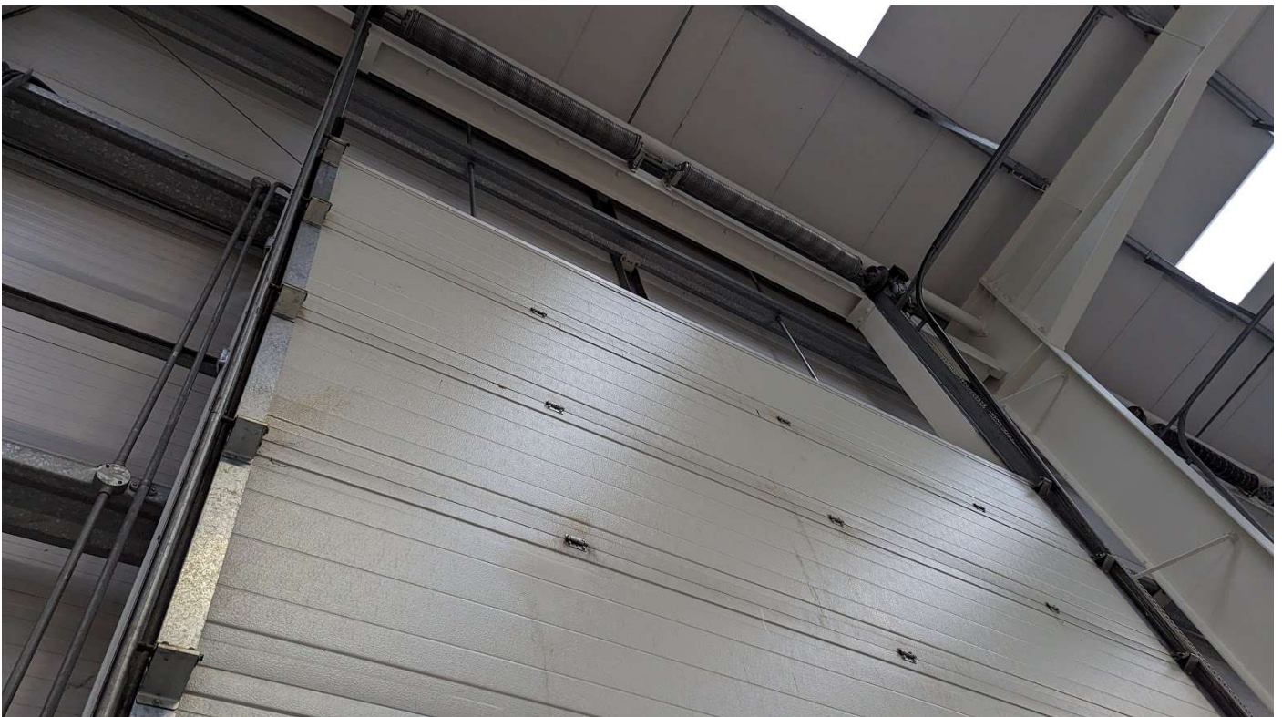
Photo 4 – View of roller shutter doors.
