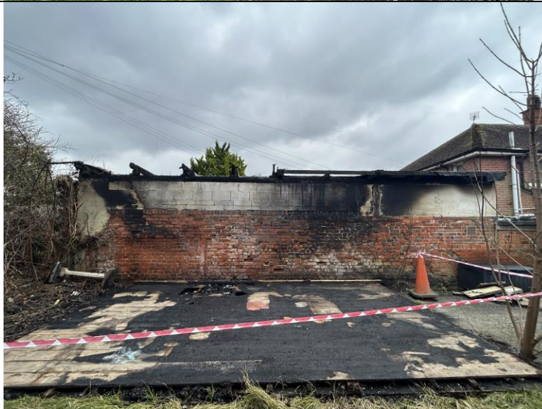
Former storage shed
