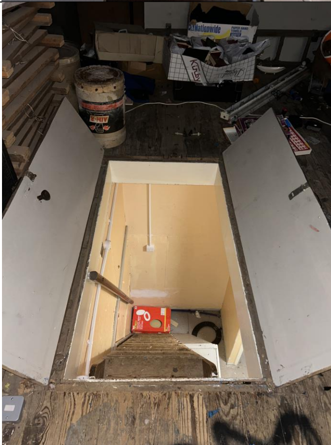
Access hatch to Mezzanine
