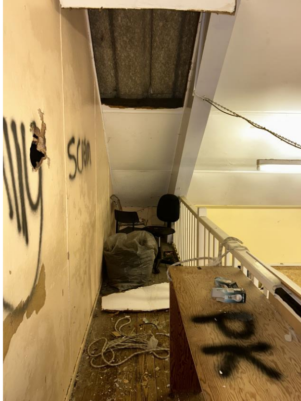
Mezzanine Balcony and Roof
