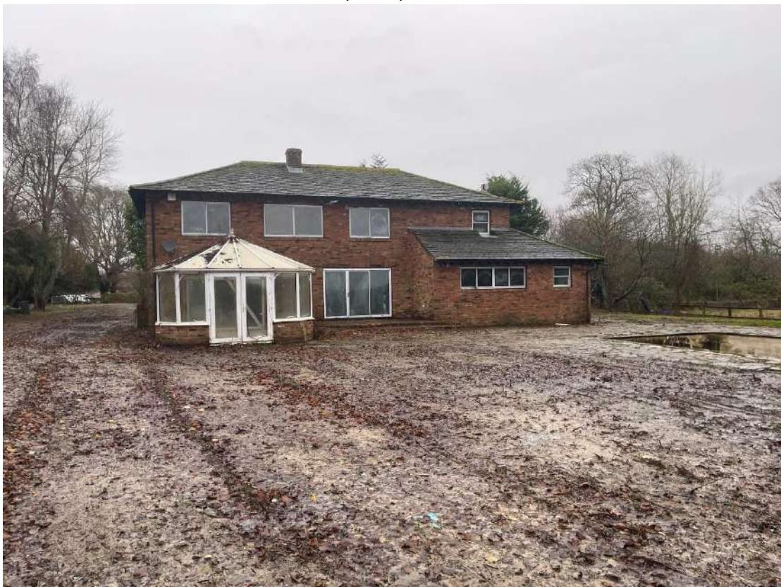
Photo2.- Jamesmead Farmhouse- Back (south) Elevation
