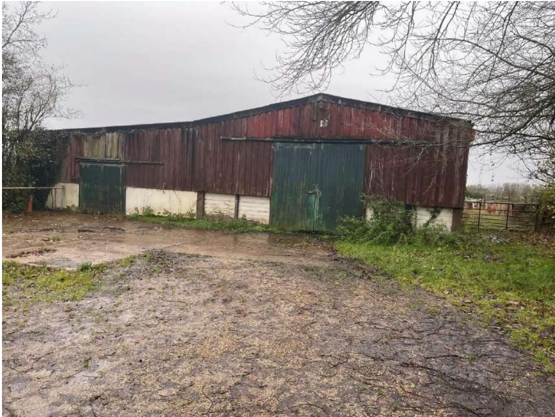
Photo 5. Main Stable Building
