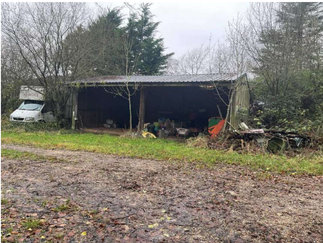
Photo 8. Open fronted store
