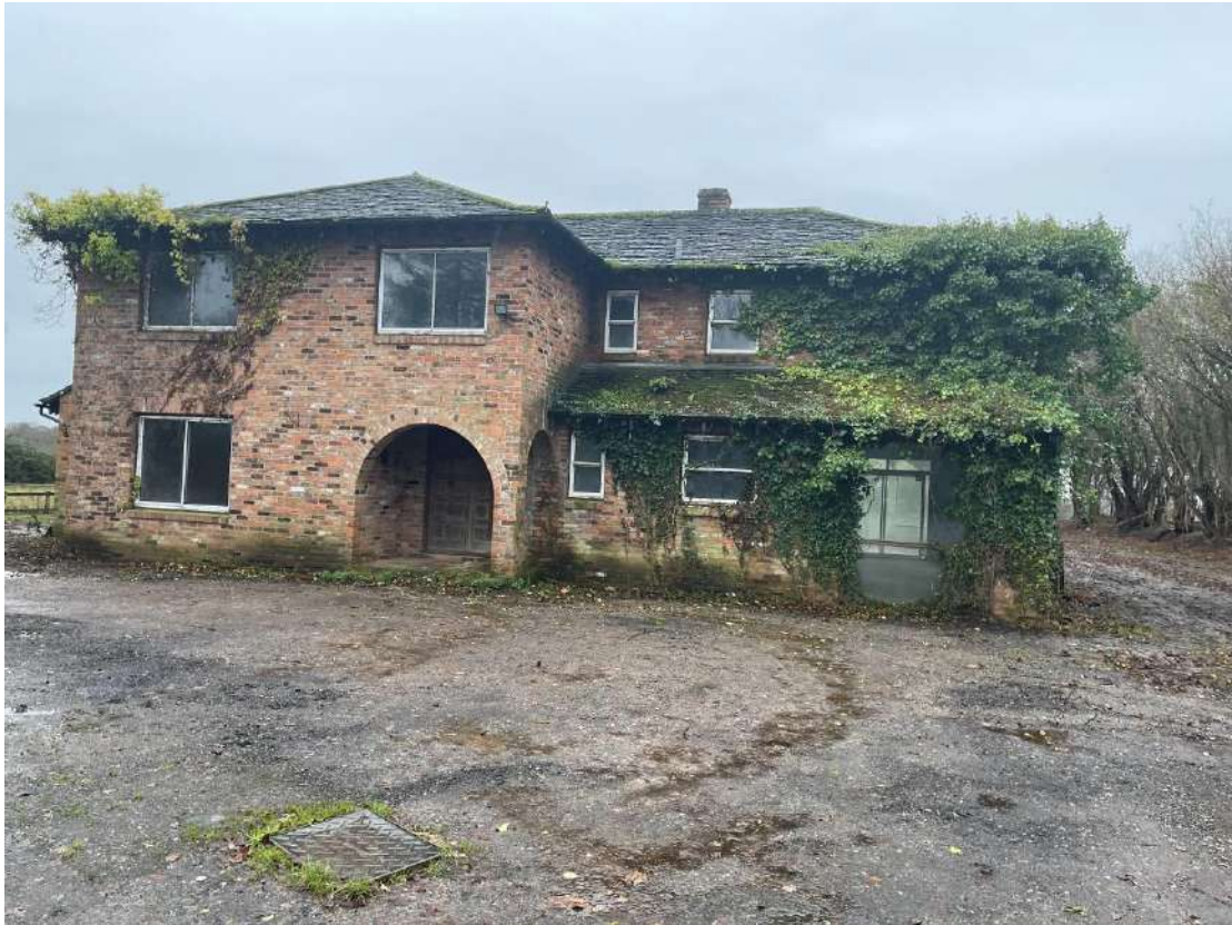
Photo 1.- Jamesmead Farmhouse- Front (North) Elevation
