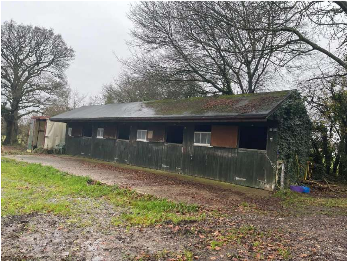
Photo 9. Timber Stable Block
