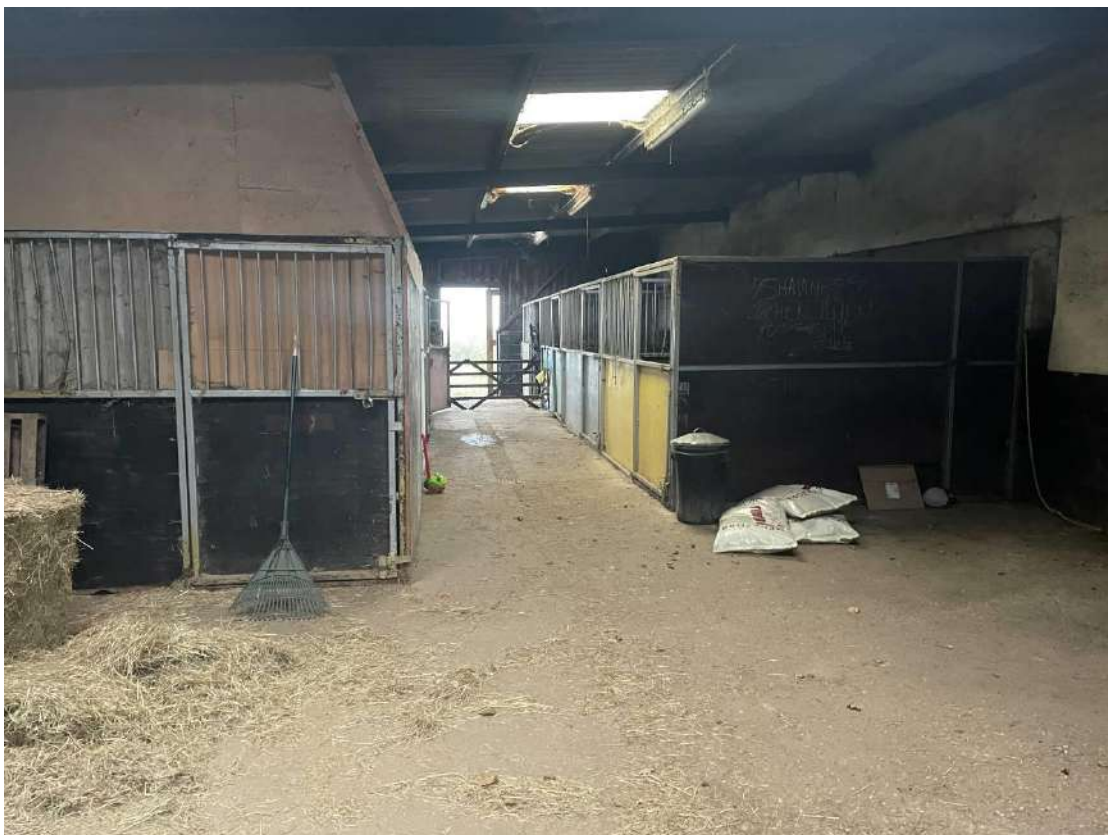
Photo 6. Internal Main Stable Building
