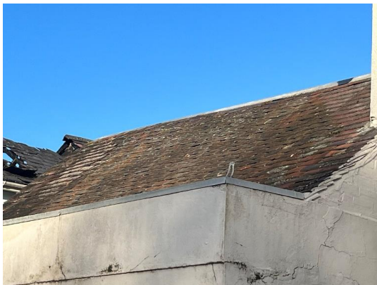
Photo 3. A section of roof on the south elevation with older tiles. Due to the age of the tiles some are damaged/ loose.
