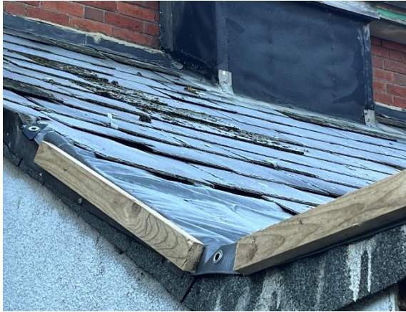
Photo 3. A section of roof on the south elevation with older tiles. Due to the age of the tiles some are damaged/ loose.
