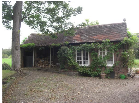
Outbuilding to be refurbished
