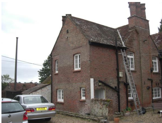
North wing facing a gravel hardstanding
