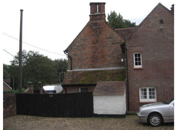
North elevation to the yard with later additions
