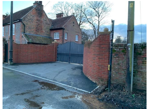
The new vehicle entrance at north end
