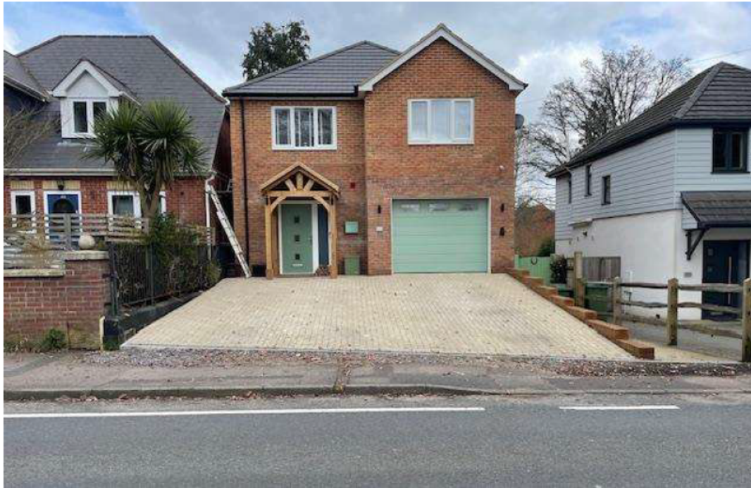
Photograph Showing the Driveway and Garage at the Application Site
