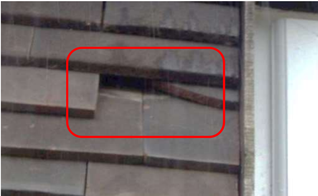
Image 7 – Evidence of gaps within the vertical hanging tiles to the dormer windows which look to offer further roosting features of value to crevice dwelling bats
