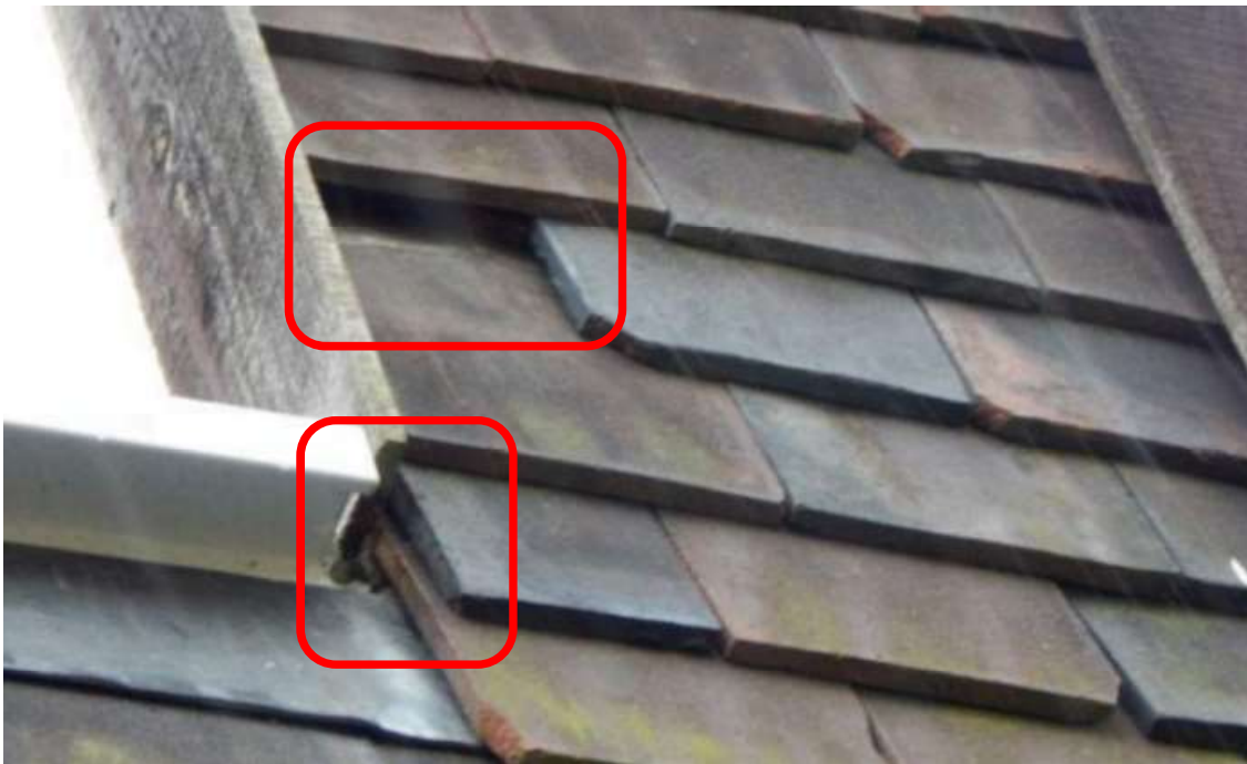
Image 6 – Evidence of gaps within the vertical hanging tiles to the dormer windows which look to offer further roosting features of value to crevice dwelling bats
