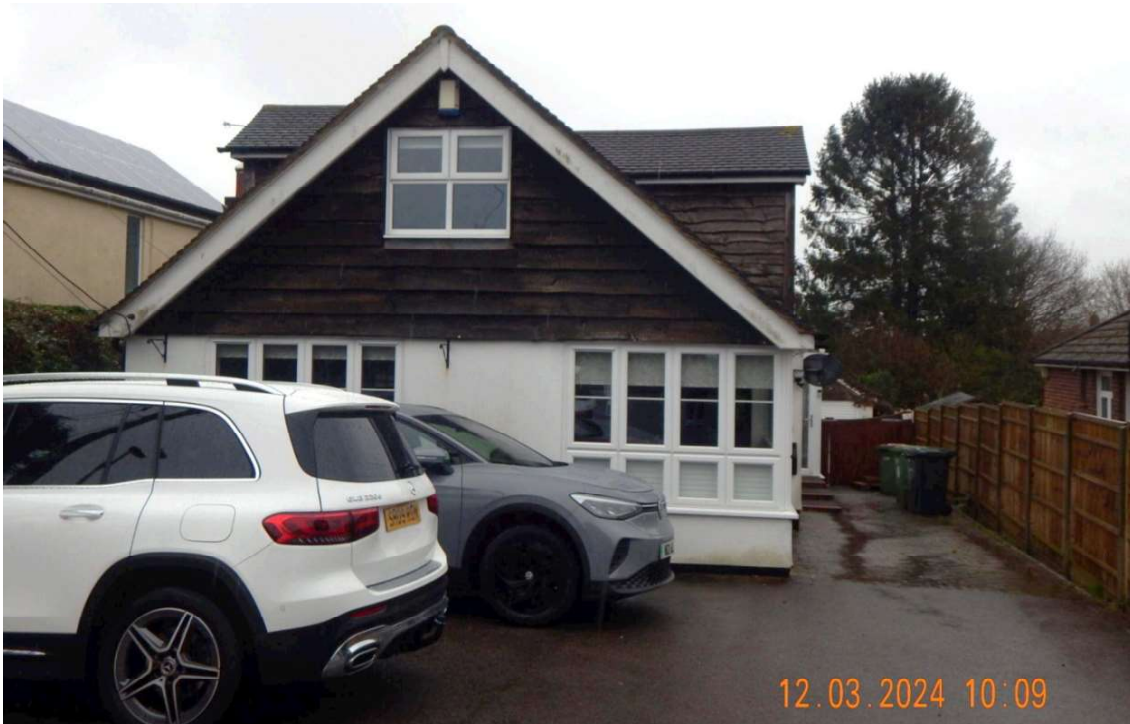
Image 1 – West facing elevation of the property
