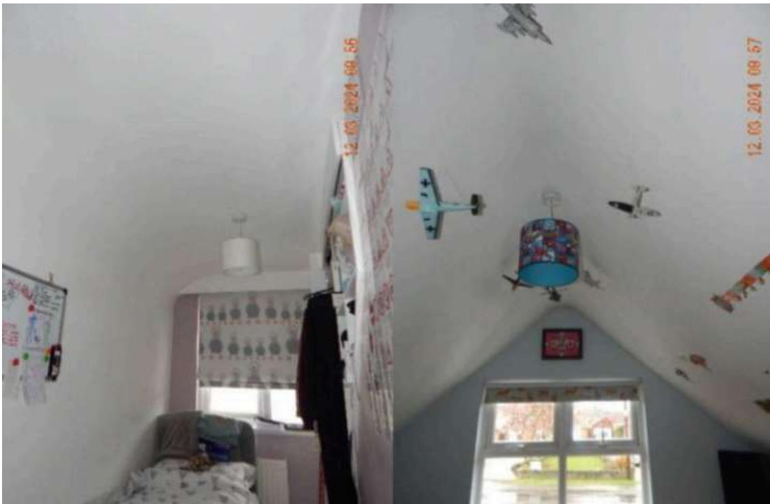
Image 8 – Internal views from within the upper floor areas of the property offering no enclosed roof void spaces
