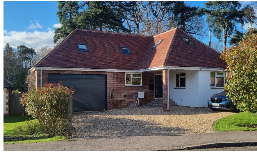
5 Thorold Road, Planning approval F/10/68006 Alterations, extension & raising of roof to create first floor habitable rooms. Flush wall/ roof side extension
