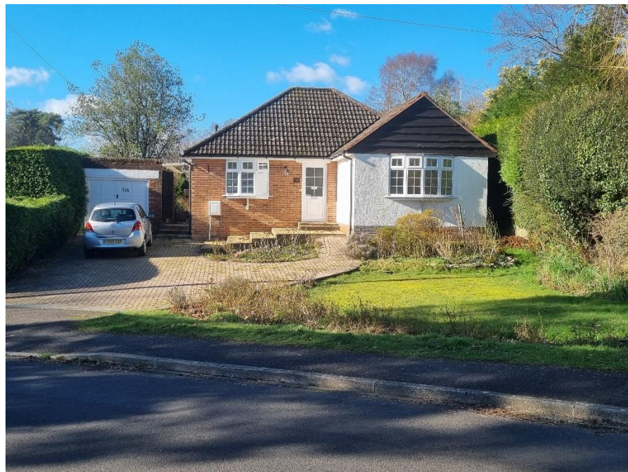
Front façade of existing dwelling facing Thorold Road.
