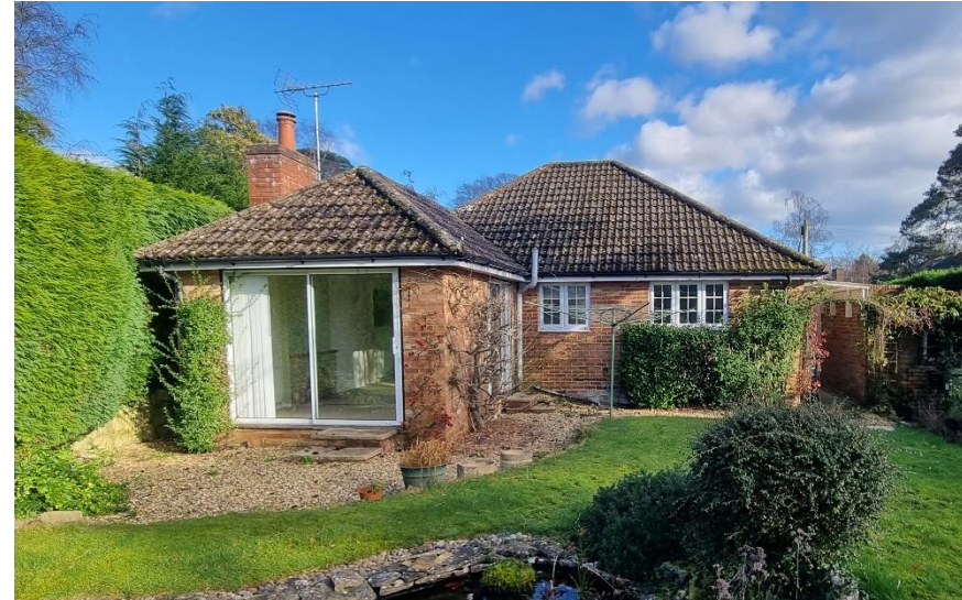
Rear façade of existing dwelling facing West.
