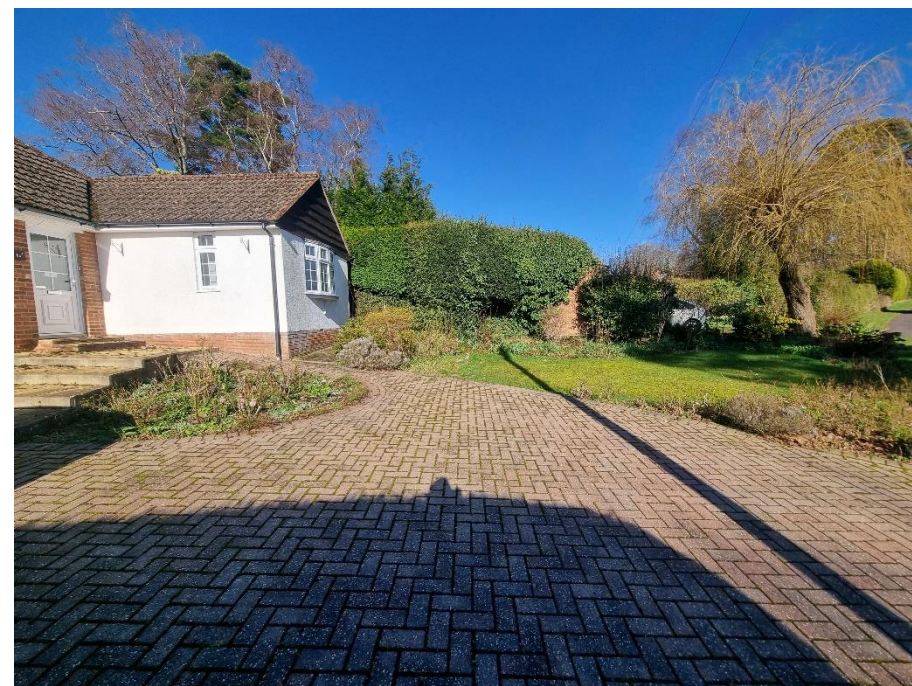
Front, North side boundary facing towards 15 Thorold Road.
