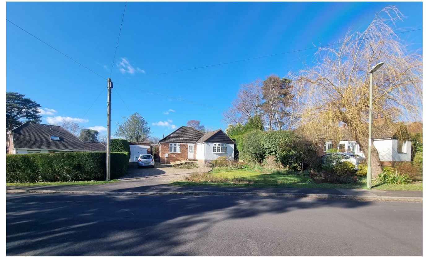
11a Thorold Road, Street scene, facing East.
