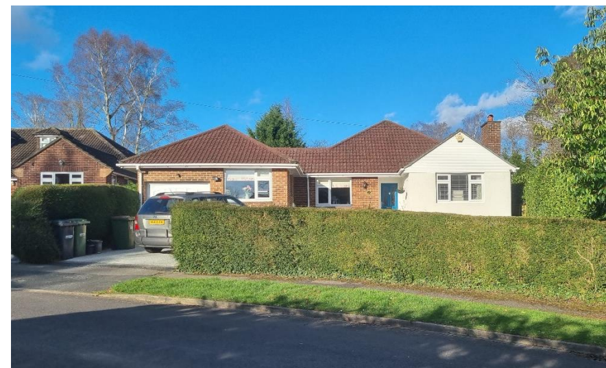
2 Heatherdene Road, planning approval Z/04851/002/00 Single storey front and rear extension. Extension pushed forward of the original building line.
