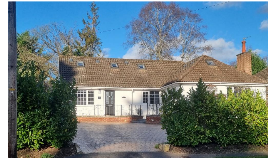
6 Heatherdene Road, planning approval Z/04770/002/00 Single storey side and rear extensions Flush wall/ gable end roof side extension.
