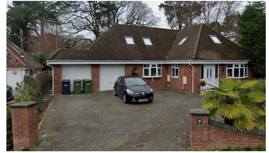
7 Thorold Road, planning approval F/07/59348 Demolition of existing to create 4 bedroom house.
