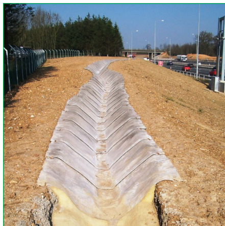
Figure 4.55 Concrete canvases (courtesy Skanska)
