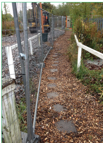
Figure 4.40 Shredded vegetation retained on site as footpath chippings (courtesy BAM Nuttall)
