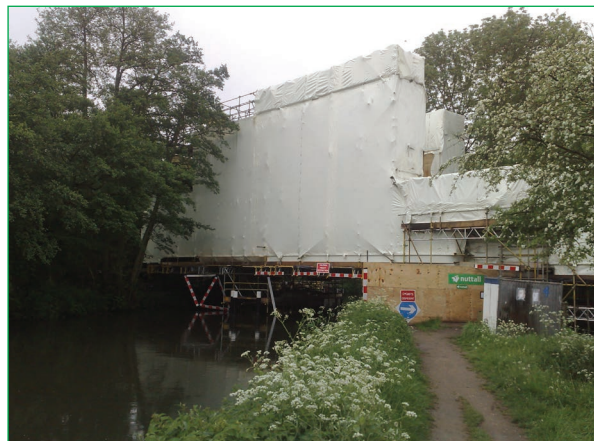
Figure 4.66 Encapsulation of blasting works (courtesy BAM Nuttall)
