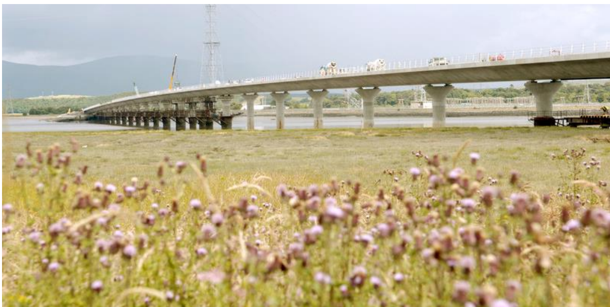
Bridge maintenance (courtesy of SEPA)
