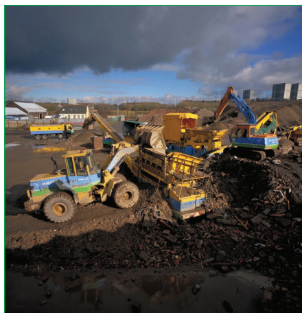
Figure 4.46 Site recycling (courtesy SEPA)
