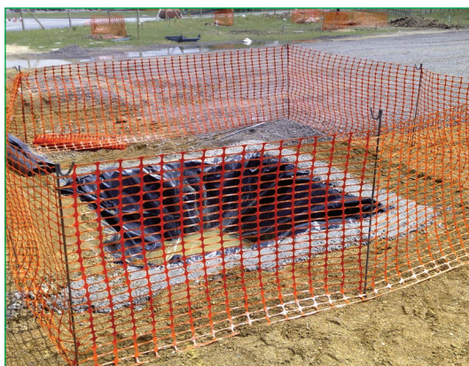
Figure 4.61 Lined washout pit (courtesy BAM Nuttall)
