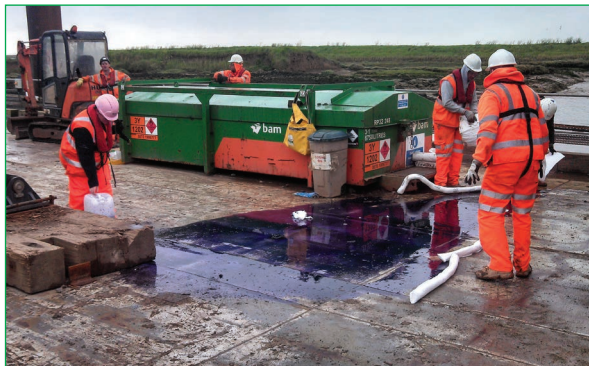
Figure 3.3 Spill drill training (courtesy BAM Nuttall)
