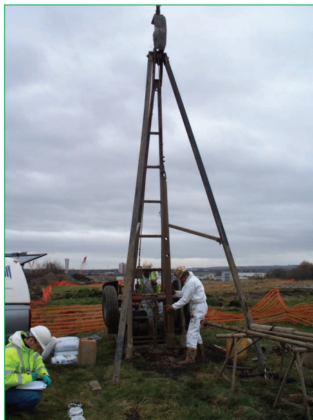
Figure 4.25 Soil testing being undertaken (courtesy Parsons Brinckerhoff)
