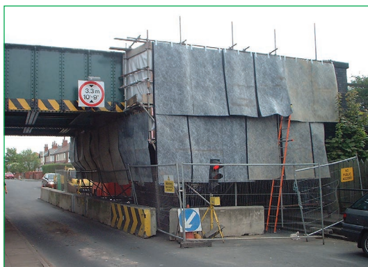
Figure 4.32 Acoustic screening (courtesy BAM Nuttall)
