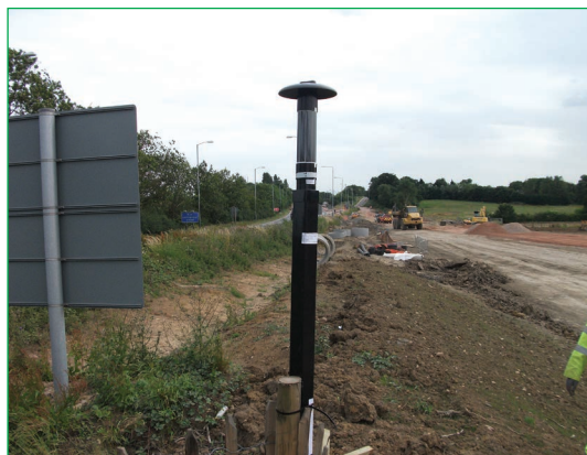
Figure 4.31 Dust monitoring (courtesy Balfour Beatty)
