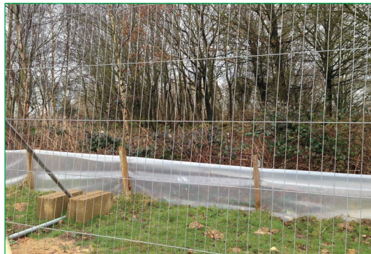
Figure 4.14 Great crested newt fencing (courtesy Brookfield Multiplex)
