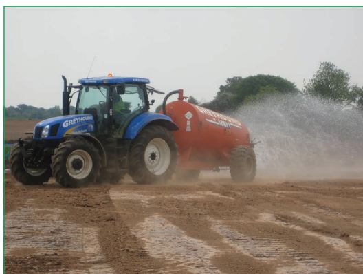
Figure 4.29 Dust suppression (courtesy Galliford Try plc)
