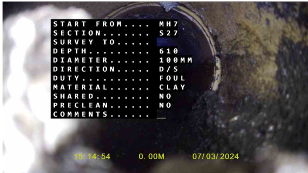
Manhole 7X_9ac00fc9-7f0a-4b62-9b38-2b116a5e613f_20240320_1250 26_166.jpg, 00:00:00, 0.00 m Start node, manhole, reference: Manhole 7
