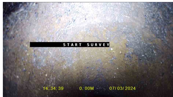
Manhole 5X_7f31e130-7087-416d-9eaa-abdc8aa46dd5_20240320_111 257_372.jpg, 00:00:03, 0.00 m Water level, 0% of the vertical dimension
