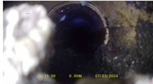
Manhole 7X_30993bdc-1365-4001-bb12-cc31c7f3c08d_20240320_125 040_456.jpg, 00:00:07, 0.00 m Water level, 0% of the vertical dimension
