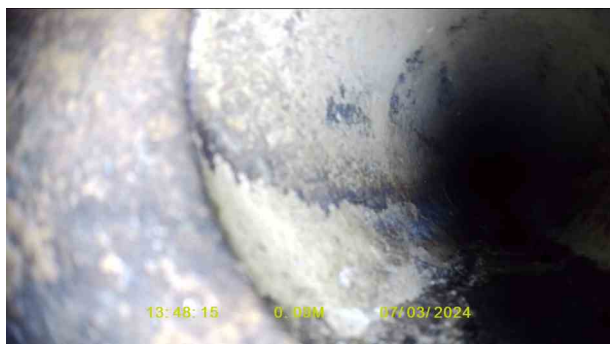
SVP 2X_e701ce62-48ed-4728-9bb5-4982212dbe85_20240320_10 0724_664.jpg, 00:00:09, 0.09 m Line deviates right
