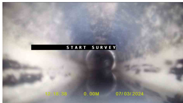
RWDP 2X_120f8a39-0d1d-448c-bfdc-e3a603941c36_20240319_154 848_226.jpg, 00:00:02, 0.00 m Water level, 5% of the vertical dimension
