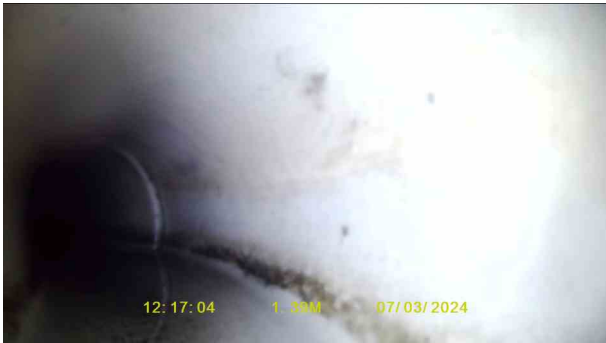
RWDP 2X_dc6a0483-51a9-48bb-8d05-fa5d8060842a_20240319_154 926_239.jpg, 00:00:29, 1.39 m Line deviates left
