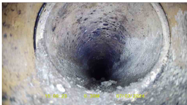
SVP 7X_efdaccdd-08b8-4519-a31f-c7a016f1bbbc9_20240320_1241 50_253.jpg, 00:00:13, 0.30 m Open joint, medium
