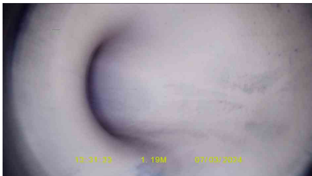
RWDP 6X_2365787b-1275-45ba-a88b-d780263c10a4_20240320_09 4057_890.jpg, 00:00:24, 1.19 m Line deviates left
