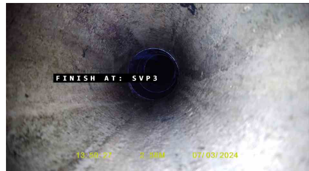
SVP 3X_764482d2-3d2c-42e2-a294-b01bbf186412_20240320_102 102_830.jpg, 00:00:54, 2.58 m Finish node, major connection without manhole, reference: SVP 3
