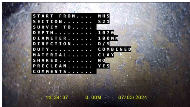
Manhole 5X_530cef70-be3e-440a-9d25-853f99eda5e4_20240320_111 247_924.jpg, 00:00:00, 0.00 m Start node, manhole, reference: Manhole 5
