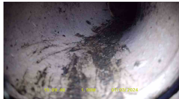
RedundantX_c8767487-f8e0-44a2-9499-a46fabd9522c_2024 0320_124639_995.jpg, 00:00:22, 1.00 m Line deviates right
