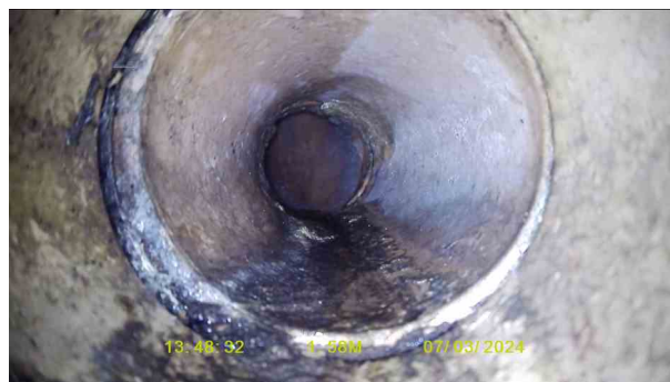
SVP 2X_a88911fc-7bdd-4968-9c5c-85725a0da2c7_20240320_100 809_241.jpg, 00:00:26, 1.49 m Open joint, medium
