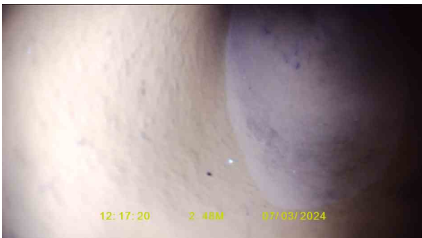
RWDP 2X_9c0cc65e-a9fc-46f7-ae64-2f922dedc7a6_20240319_1550 30_885.jpg, 00:00:45, 2.48 m Line deviates up, Rest Bend
