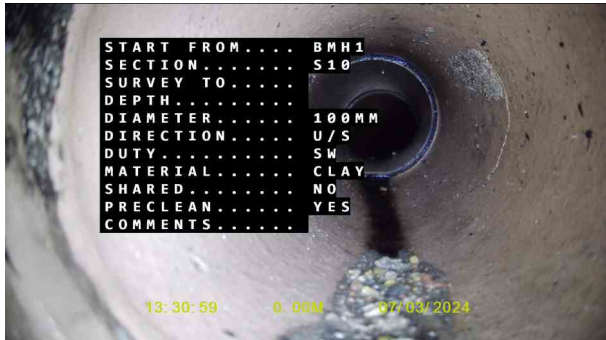
RWDP 6X_48c3c450-ee51-428c-853e-b610d2734ff1_20240320_093 559_831.jpg, 00:00:00, 0.00 m Start node, manhole, reference: Buried MH
