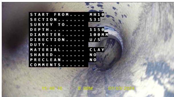
RedundantX_19581056-f0ce-4593-a567-1ac8569a34a2_2024 0320_134210_883.jpg, 00:00:00, 0.00 m Start node, manhole, reference: Manhole 10
