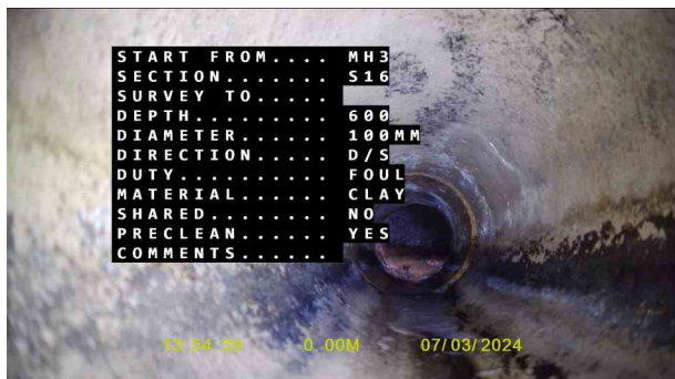
Manhole 3X_12842336-abf2-45fb-84b0-83f78cc49ba8_20240320_1036 28_451.jpg, 00:00:00, 0.00 m Start node, manhole, reference: Manhole 3
