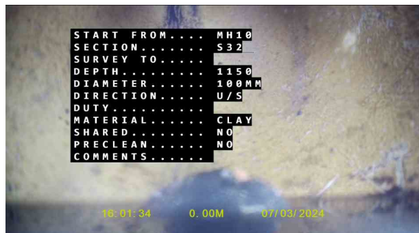
RedundantX_ffe9b83d-0ebd-414b-a04f-fb2861c169c9_2024 320_134554_297.jpg, 00:00:00, 0.00 m Start node, manhole, reference: Manhole 10
