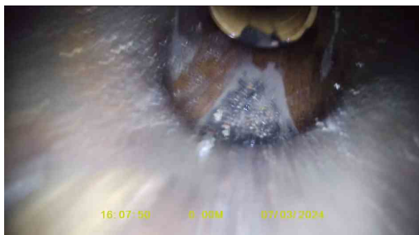
Manhole 10X_edd32b4f-5ecd-478b-b1df-b00fcd28c93c_20240320_135 340_224.jpg, 00:00:11, 0.10 m General remark, Drops into main channel
