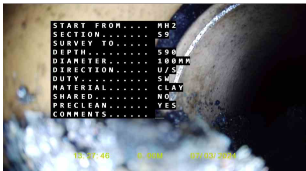
Buried MHX_88f816ba-bc89-4922-bad5-ee9d8fa42103_20240319_172343_632.jpg, 00:00:00, 0.00 m Start node, manhole, reference: Manhole 2
