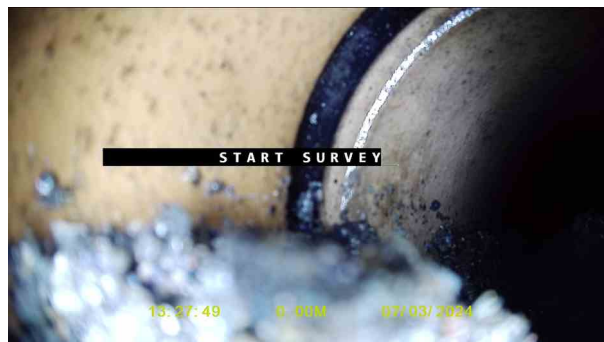
Buried MHX_b9240e3f-b9a0-4f84-bd62-2fc018511bbe_20240319_172406_020.jpg, 00:00:03, 0.00 m Water level, 0% of the vertical dimension
