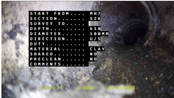
RedundantX_ee872050-97e9-48db-a77a-5383d729ed70_202 40320_124539_411.jpg, 00:00:00, 0.00 m Start node, manhole, reference: Manhole 7
