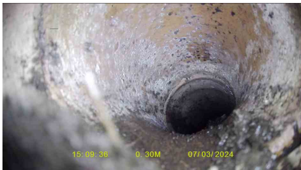
RedundantX_bfcb4812-3e59-4124-8a38-283a3c0081ef_2024 0320_124609_171.jpg, 00:00:11, 0.30 m Line deviates right
