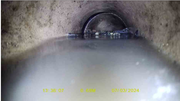
Manhole 2X_e180e7ba-86a9-4a04-bb00-ab7548002c6b_20240320_095628_250.jpg, 00:00:16, 0.69 m Water level, 30% of the vertical dimension
