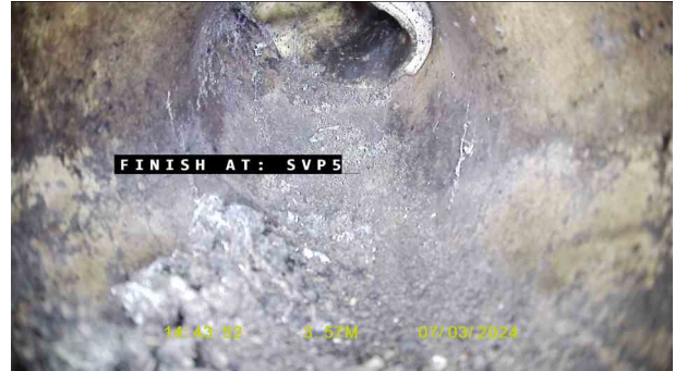
SVP 5X_ccf33f04-5cb7-4e05-a1c5-17635955b5bf_20240320_1124 17_278.jpg, 00:01:05, 3.57 m Finish node, major connection without manhole, reference: SVP 5
