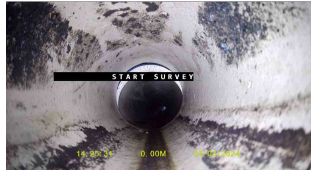
Manhole 4X_f07848c6-1dfe-4669-8032-c440a459f597_20240320_104317_089.jpg, 00:00:03, 0.00 m Water level, 0% of the vertical dimension
