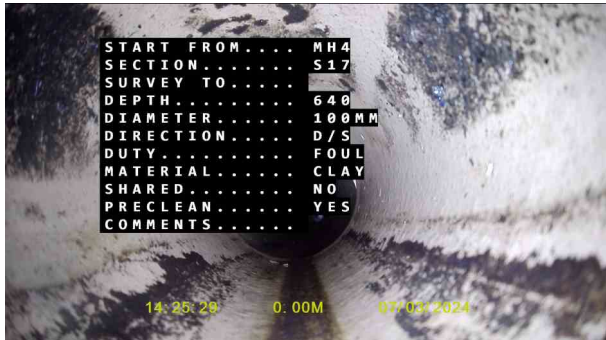
Manhole 4X_2e843ea6-c5e3-4873-839c-892c0a61098a_20240320_104306_183.jpg, 00:00:00, 0.00 m Start node, manhole, reference: Manhole 4
