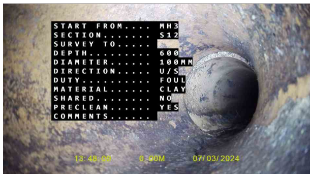
SVP 2X_5b7a163b-cae7-4a54-9598-d4a6872b6c92_20240320_10 0647_734.jpg, 00:00:00, 0.00 m Start node, manhole, reference: Manhole 3
