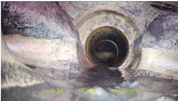
Manhole 1X_245adb34-42d7-4e86-a80d-f83f5ad719d1_20240319_163522_052.jpg, 00:03:26, 10.53 m Finish node, manhole, reference: Manhole 2
