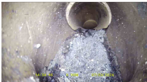
Manhole 5X_58e5fa59-be5e-434e-8fd9-ab32cc1e031b_20240320_111 348_530.jpg, 00:00:10, 0.10 m General remark, Drops into main channel
