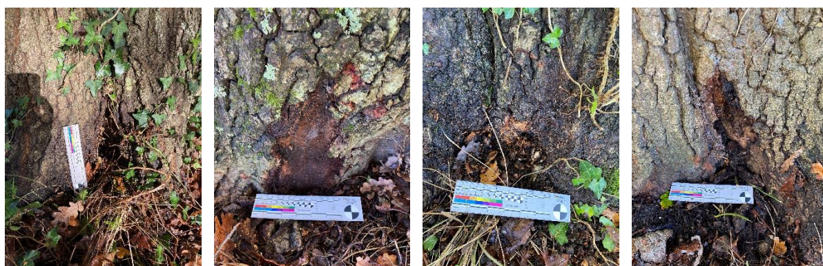
SAL6, 7, 8 and 9 T3 with loose bark and cavity formation at the base.
