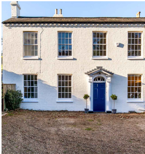
3 - Old Rectory 19th century rectory previously servicing St Marys Church to the north.
