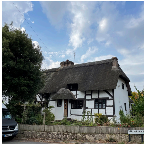
5 - 117 & 119 Spring Lane 16th century timber-framed thatched house, split into two dwellings.
