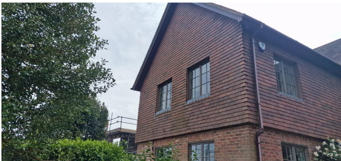
Picture 2: Showing the front elevation of the building.
