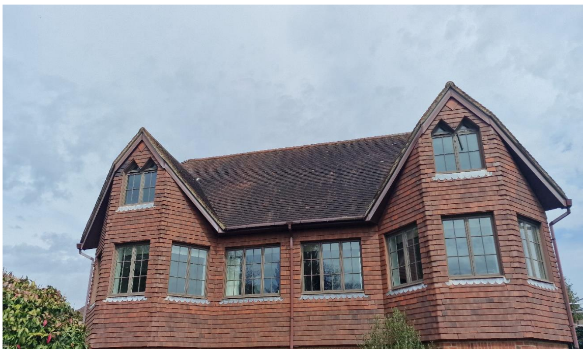
Picture 3: Showing the rear of the building.
