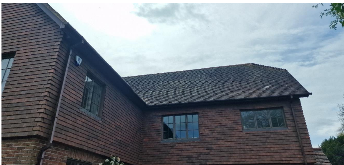
Picture 1: The front elevation showing the roof and hanging tiles.
