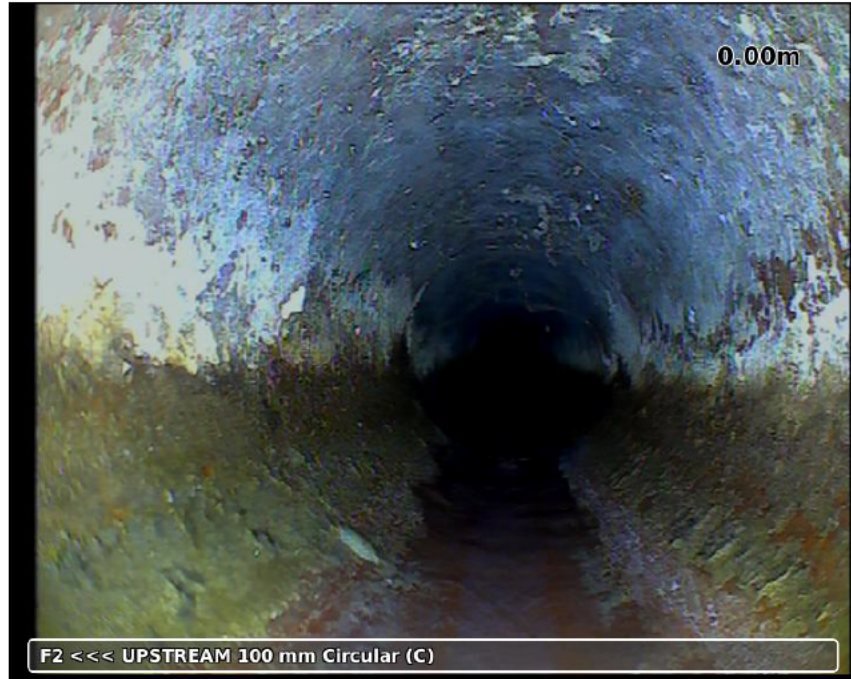
Photo: 20230130-083212-snap0000.jpg, 00:00:04 0m, Start node type manhole reference number: F2
