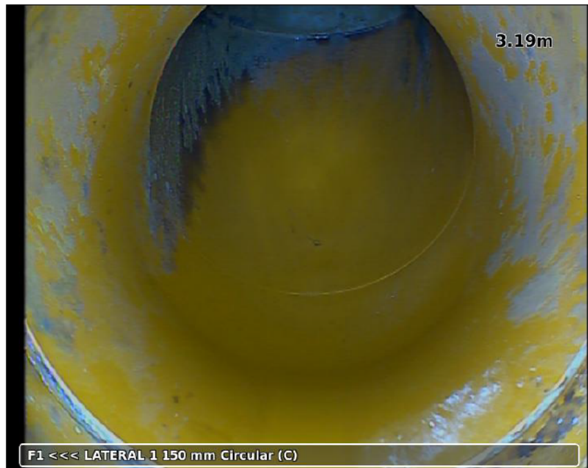
Photo: 20230130-082242-snap0001.jpg, 00:00:58 3.19m, Finish node type outfall reference number: LATERAL 1 INTERNAL WASTE STACK
