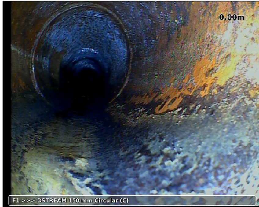
Photo: 20230130-082748-snap0000.jpg, 00:00:02 0m, Start node type manhole reference number: F1
