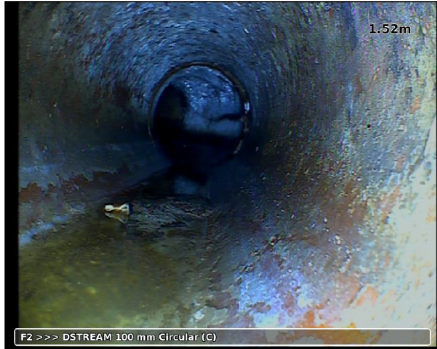
Photo: 20230130-083451-snap0004.jpg, 00:01:36 1.52m, Size changes new size(s) 150 mm high 150 mm wide
