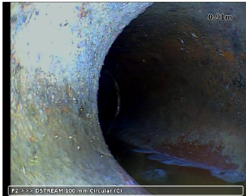
Photo: 20230130-083451-snap0003.jpg, 00:01:17 0.91m, Line deviates left Remarks: DROPPING INTO PIPE RUNNING FROM MANHOLE F1
