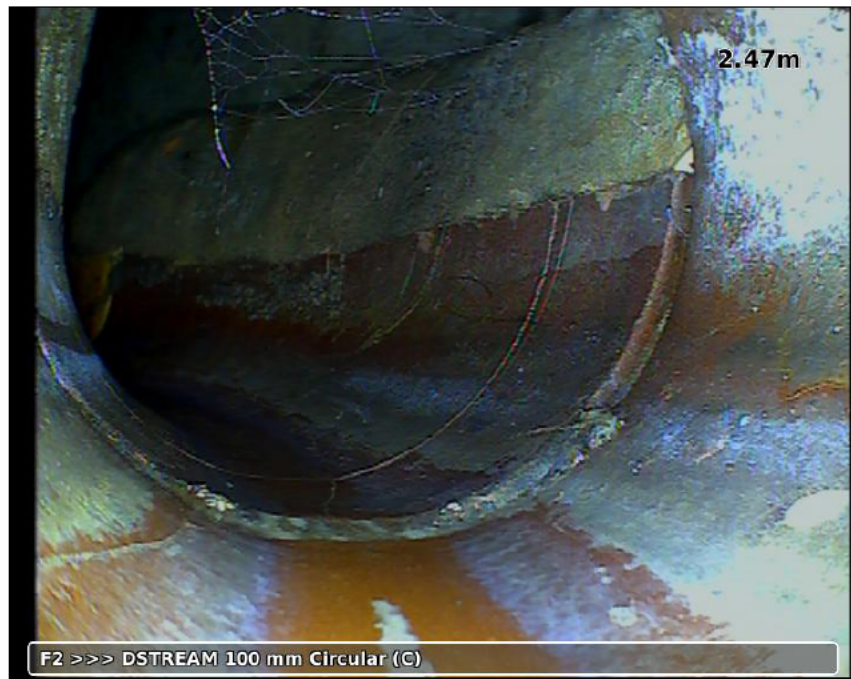
Photo: 20230130-083451-snap0005.jpg, 00:01:56 2.47m, Line deviates left
