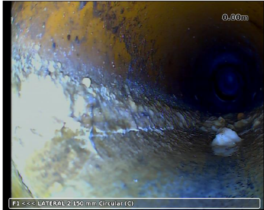
Photo: 20230130-082500-snap0000.jpg, 00:00:01 0m, Start node type manhole reference number: F1
