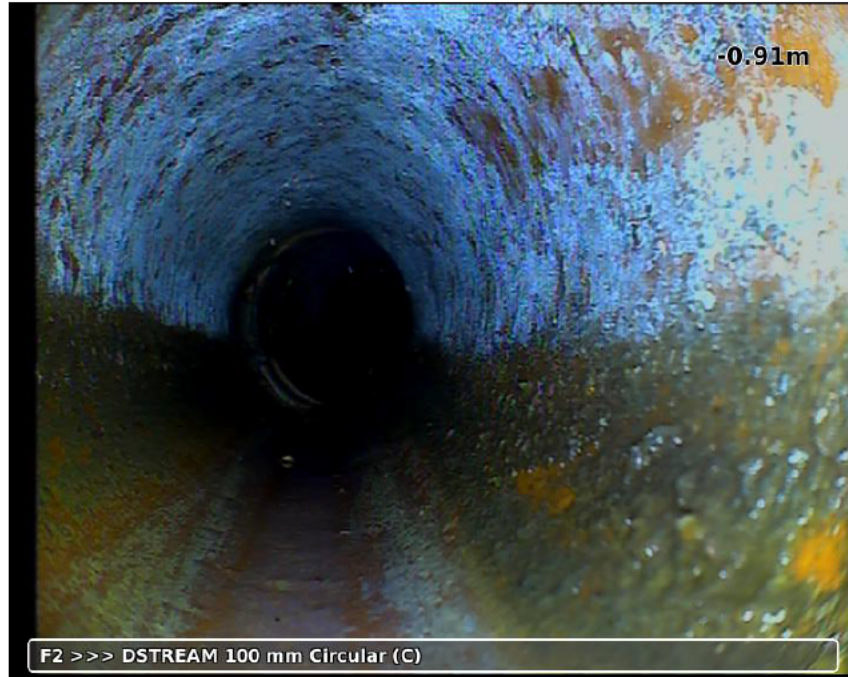
Photo: 20230130-083451-snap0000.jpg, 00:00:00 -0.91m, Start node type manhole reference number: F2
