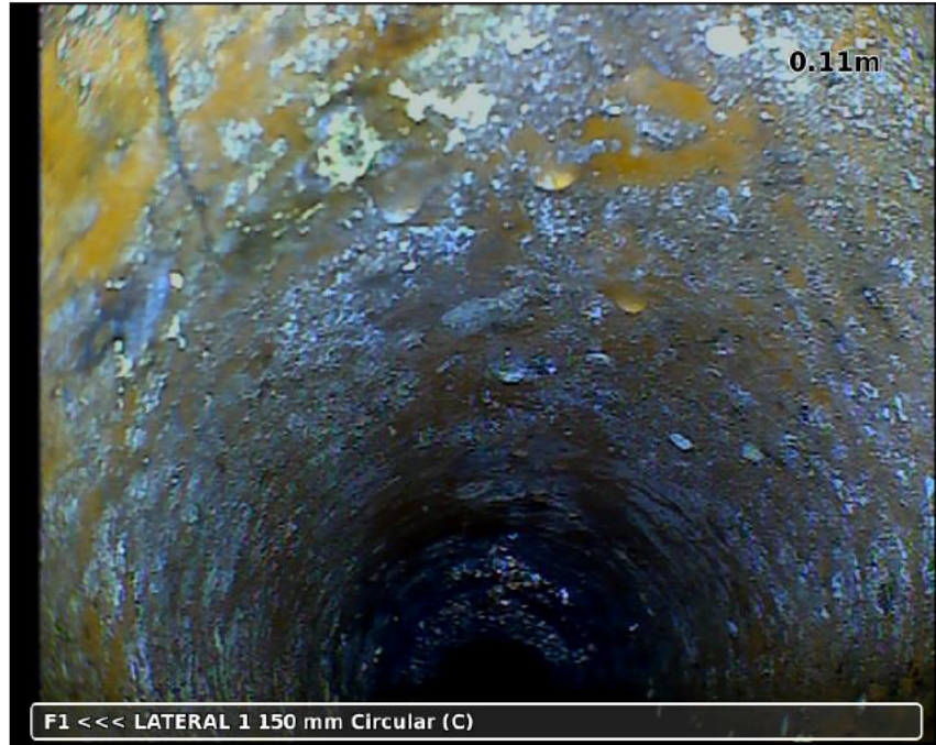
Photo: 20230130-082242-snap0000.jpg, 00:00:07 0.11m, Start node type manhole reference number: F1
