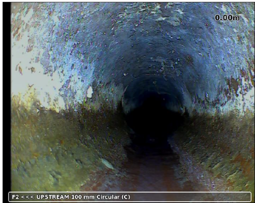
Photo: 20230130-083212-snap0001.jpg, 00:00:07 0m, Water level 05 % of the vertical dimension
