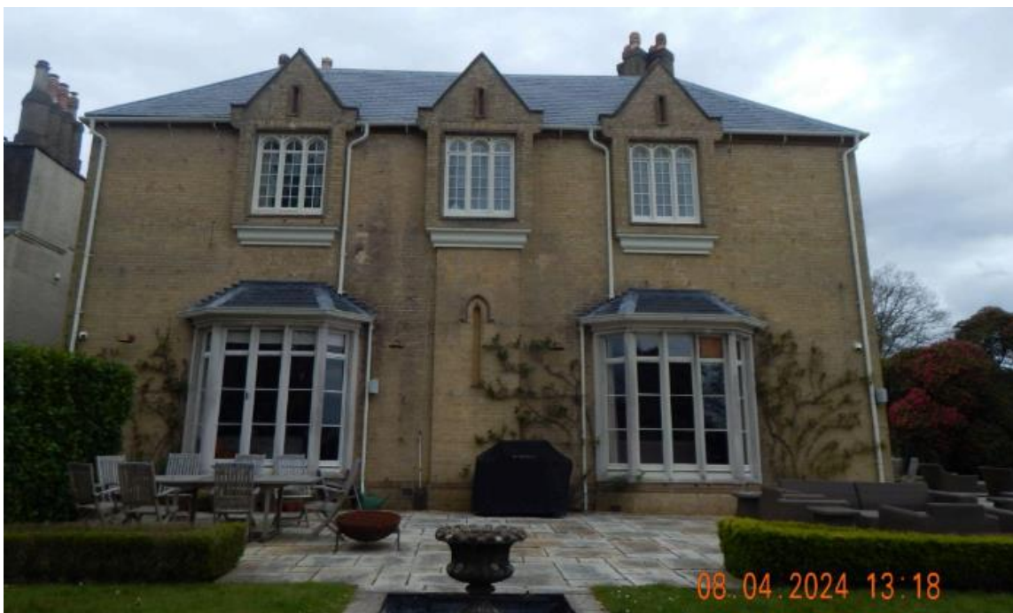
Image 2 – South facing elevation of the main dwelling
