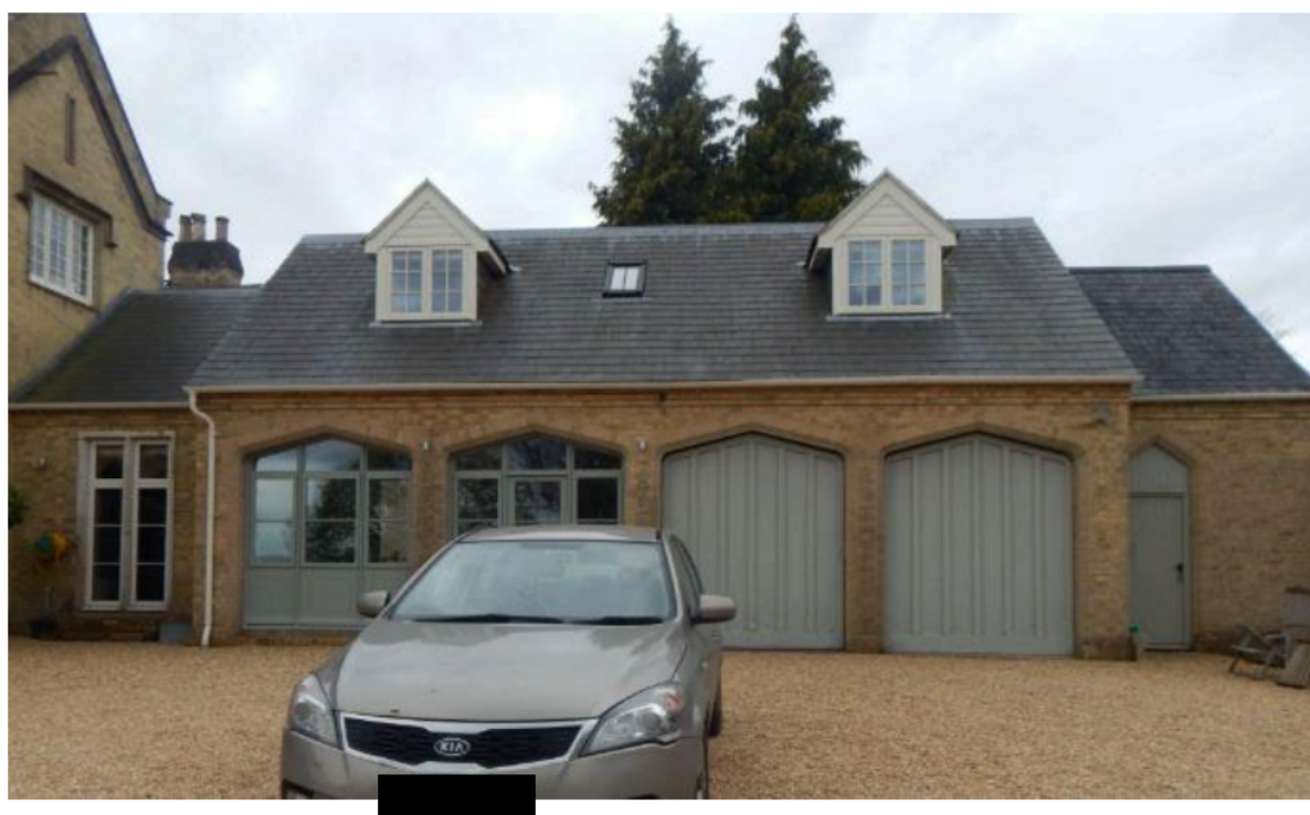
Image 9 – East facing elevation of the garage/annex structure
