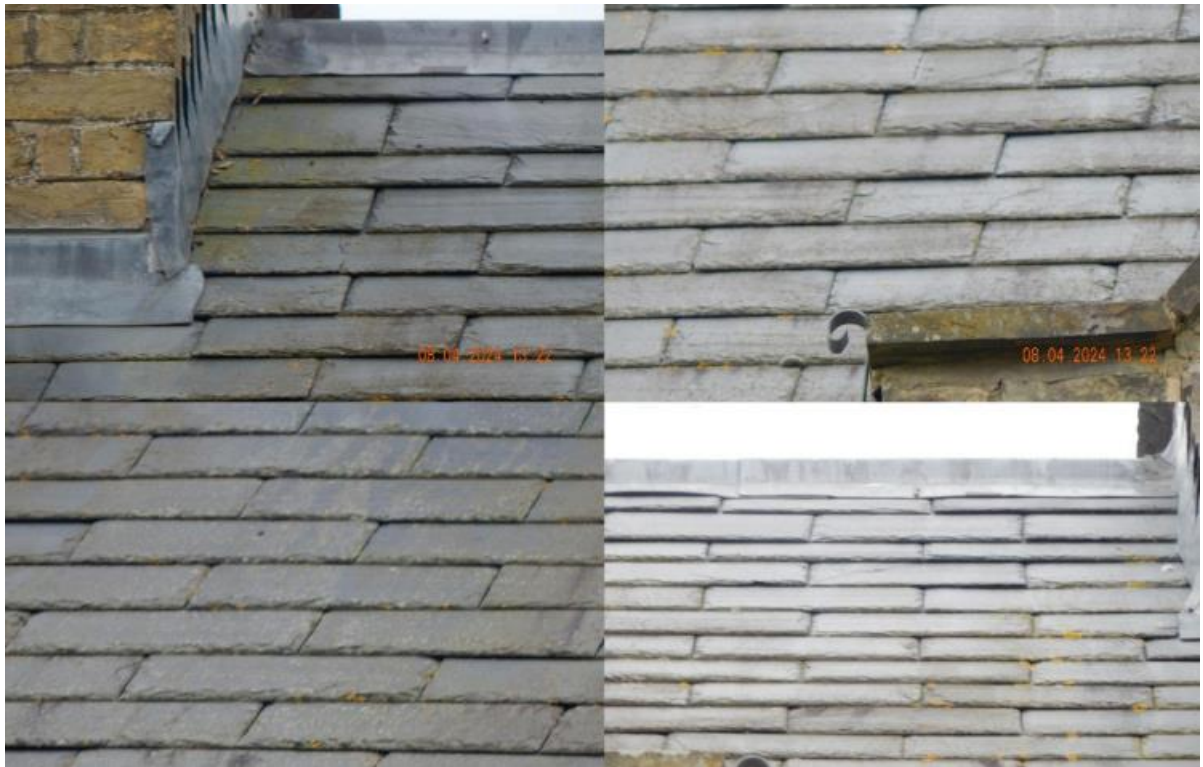
Image 5 – Example image of main roof coverings which have demonstrated a well-maintained covering throughout
