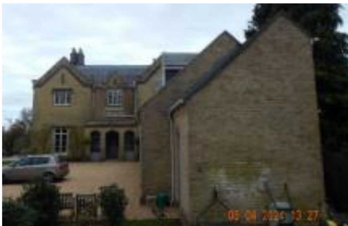
Image 10 – North facing elevation of the garage/annex structure
