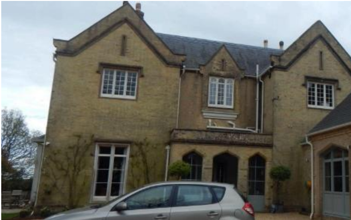
Image 1 – North facing elevation of the main dwelling
