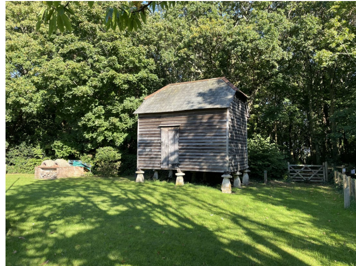
Plate 8 The granary, looking south-east
